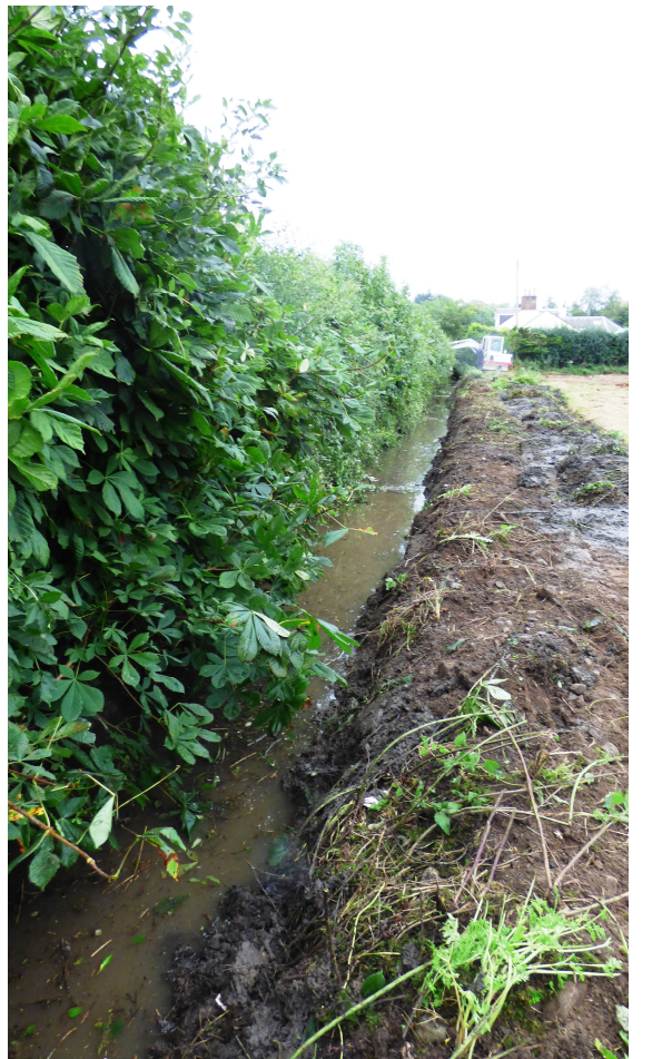
Figure 9d - ditch after clear out (WSW half)
