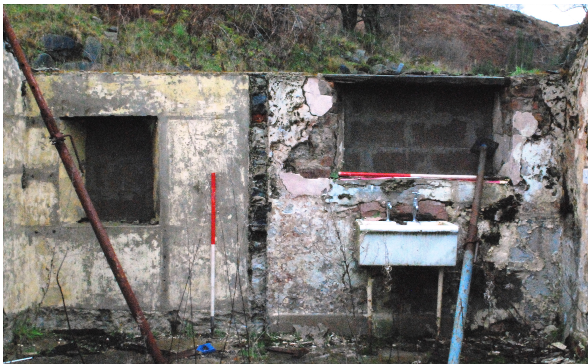
Figure 11a – N-end (small extension) of eastern (rear) elevation (from W)
