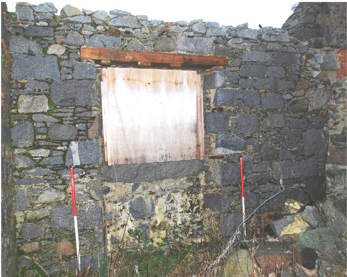
Figure 14b – southern end of western (front) elevation (interior) (from E)
