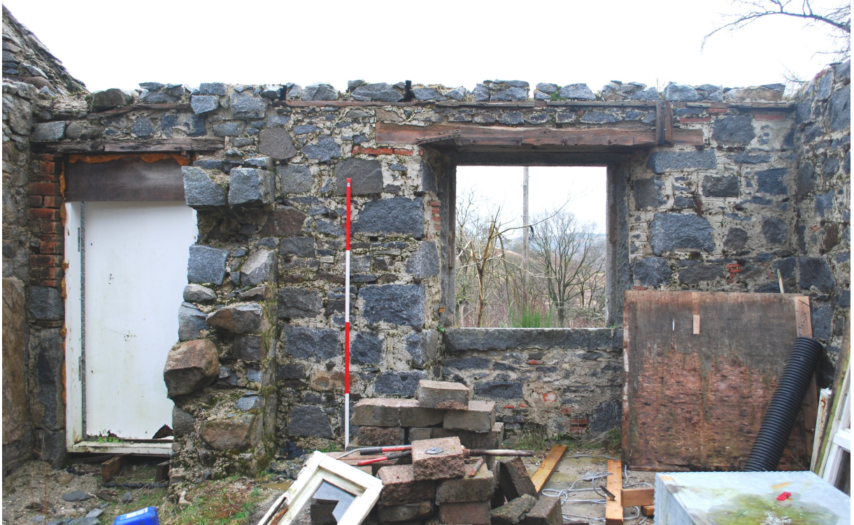
Figure 15a – western (front) elevation (northern end) (interior) (from E)
