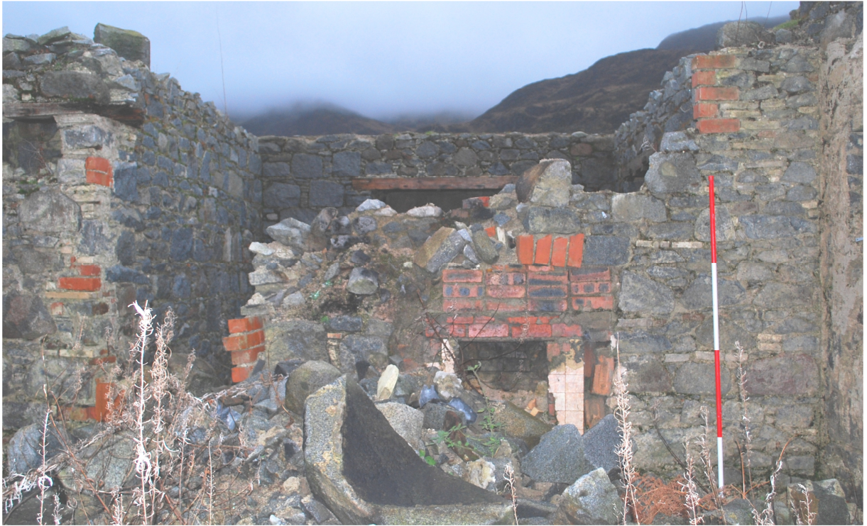
Figure 16a - dividing wall showing fireplace (see Figure 19a) (from N)
