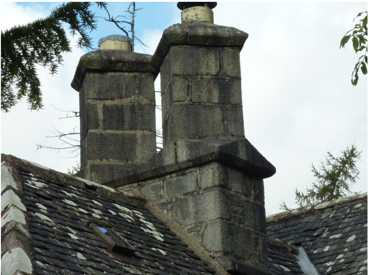
Figure 20 - chimneys in-situ (c) Andy Nicholson
