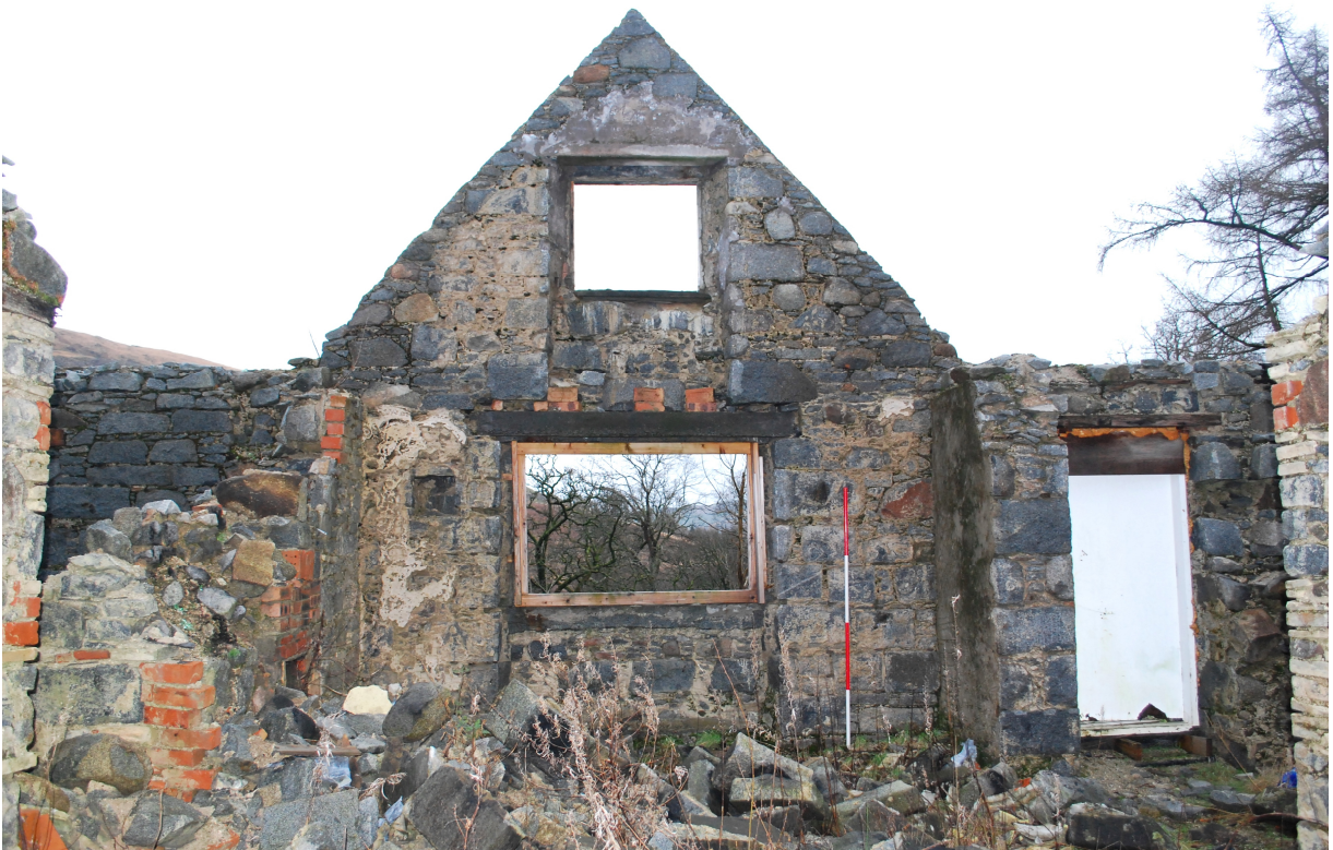
Figure 15b – western (front) elevation (central area) (interior) (from E)
