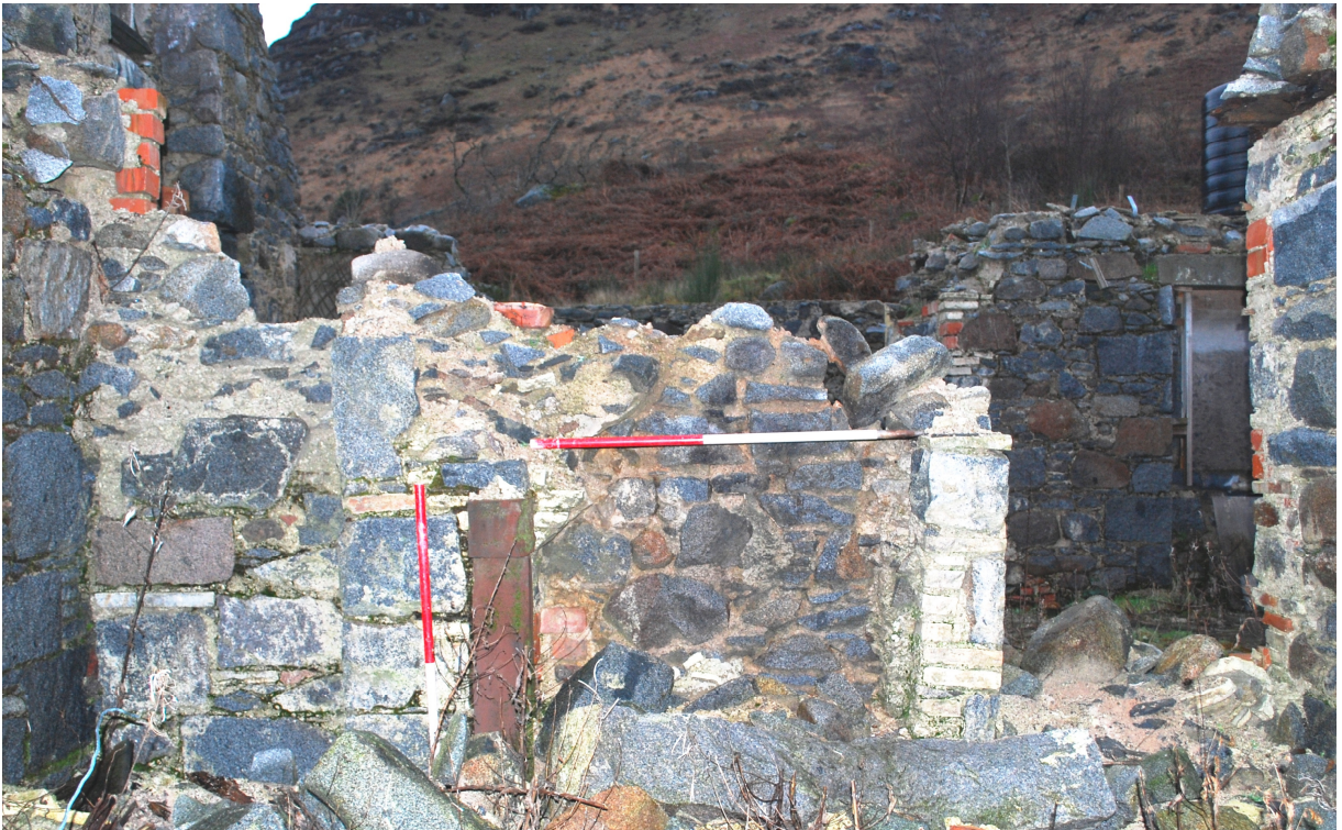
Figure 16b - dividing wall showing fireplace (see Figure 19a) (from S)
