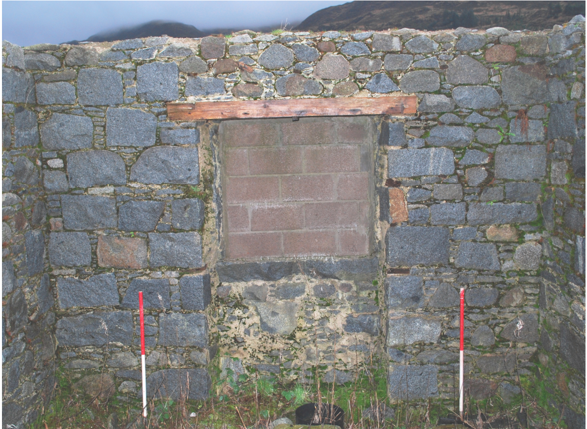
Figure 14a – southern end wall (interior) (from N)
