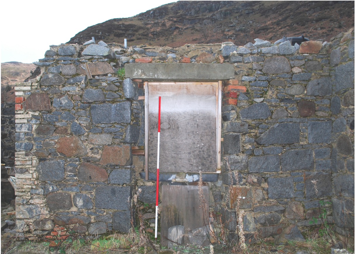
Figure 13a – N-wall of later extension (see Figures 19-b) (from S)
