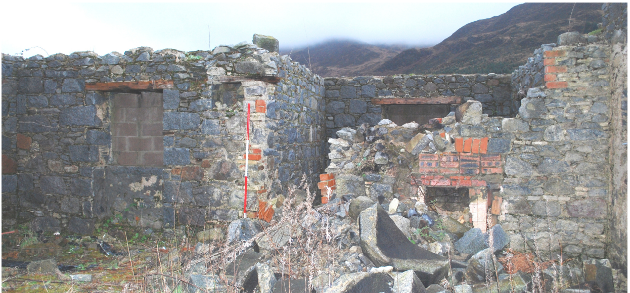
Figure 17b - internal dividing wall containing fireplaces (from N)
