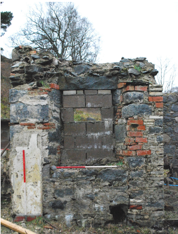
Figure 12b - later blocked-in window in E-elevation (interior) (from W)
