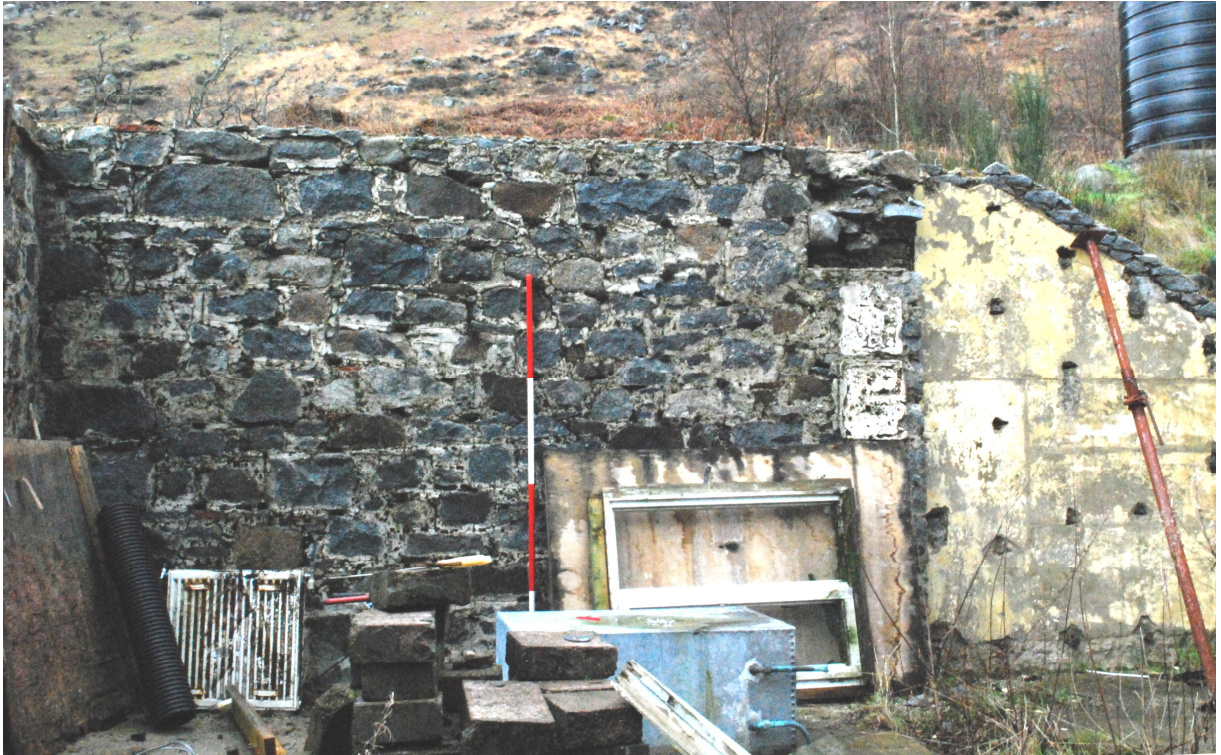
Figure 10a – northern end wall (interior) (from S)
