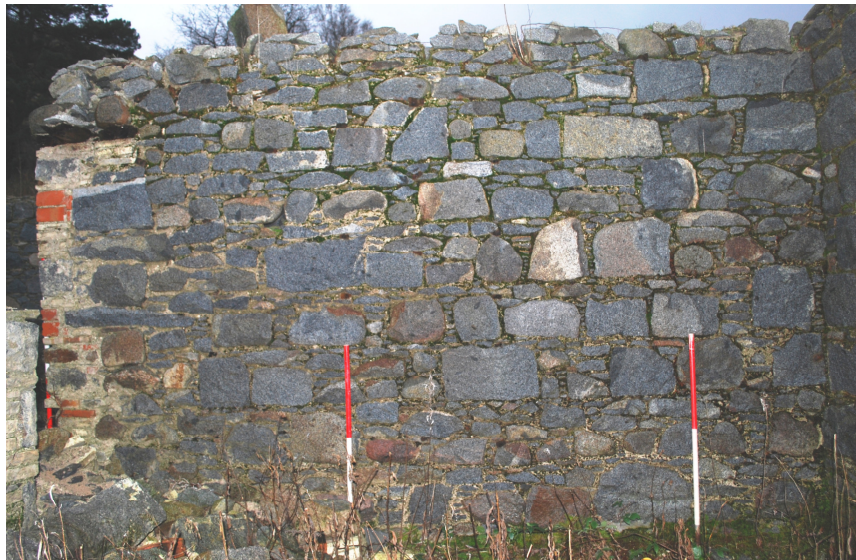
Figure 17a - southern end of eastern (rear) elevation (from W)
