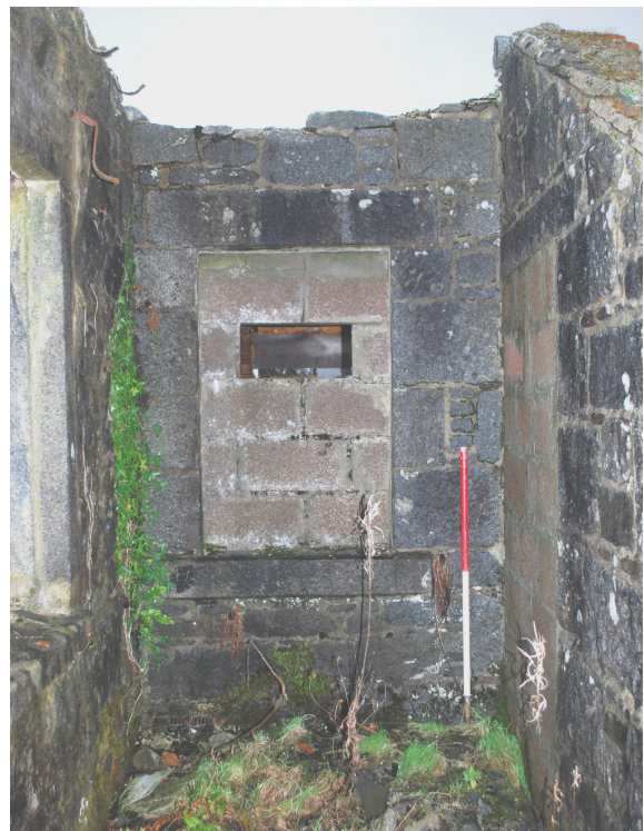
Figure 12c - later blocked-in window in E-elevation (exterior) (from E)
