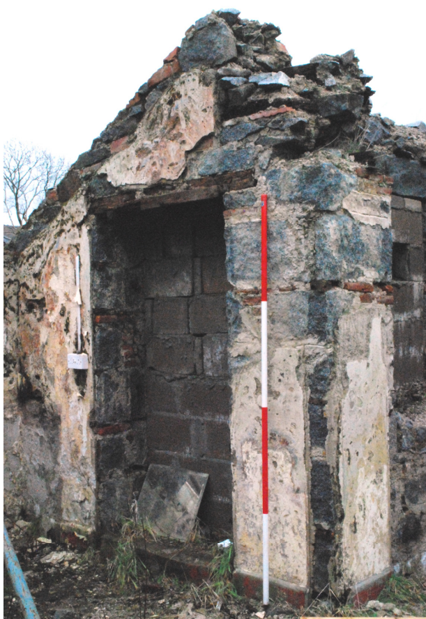
Figure 11b - S-wall of small extension showing blocked in doorway (interior) (from NNW)
