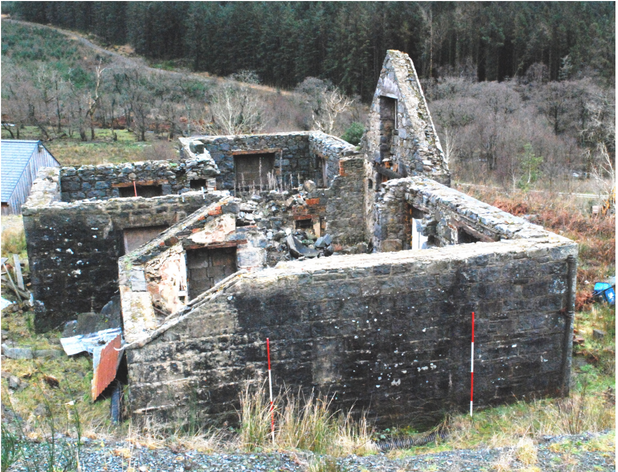
Figure 8a - general of Glenhead farm house (from NE)
