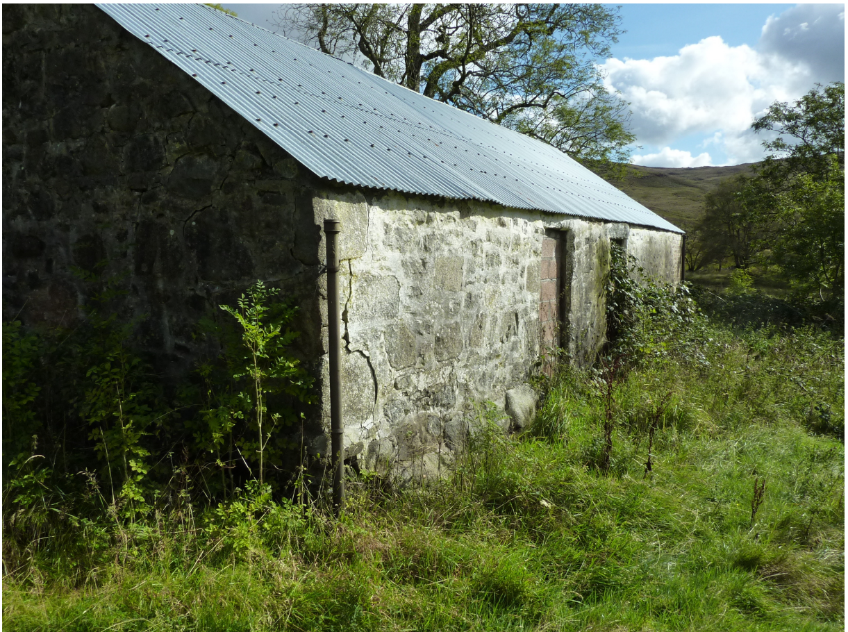
Figure 21b - original farmstead prior to demolition (c) Andy Nicholson
