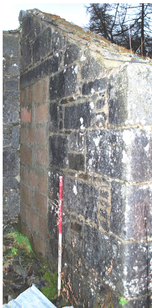
Figure 11c - S-wall of small extension showing blocked-in doorway (from ESE)
