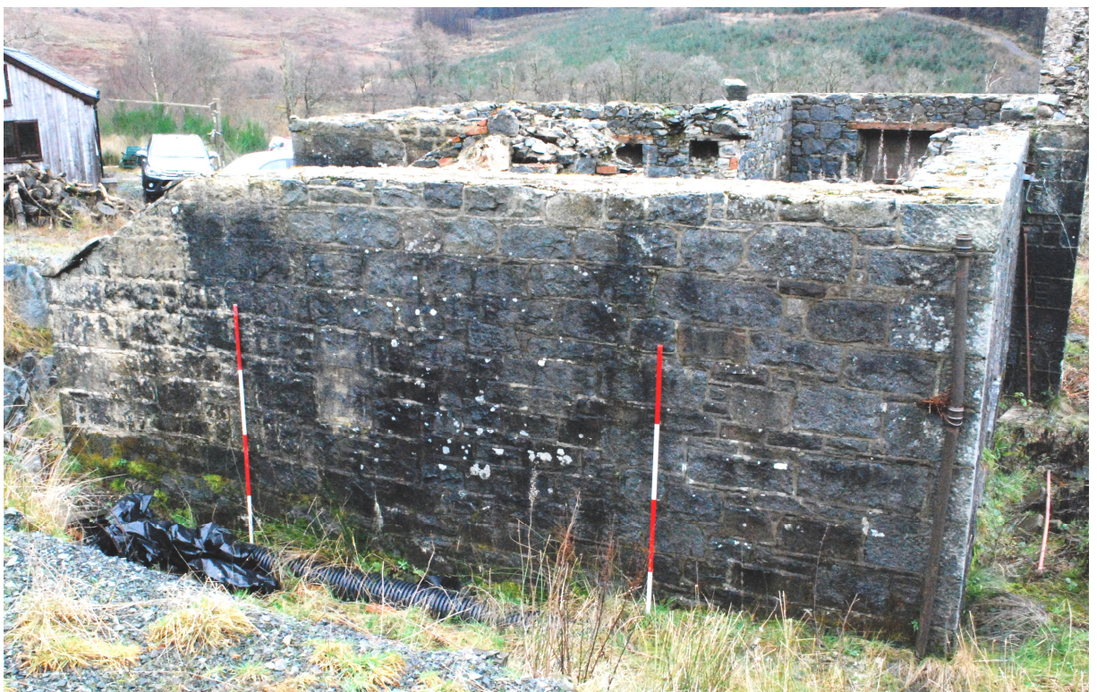
Figure 9b – northern end of Glenhead Farm House (from N)
