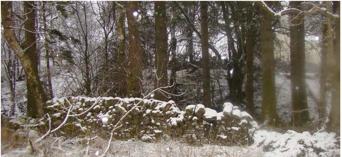
Figure 6b - old boundary wall (middle section)
