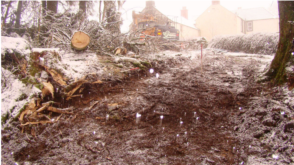
Figure 5a – post-ex image showing subsoil [102] in E / W section (from SSW)
