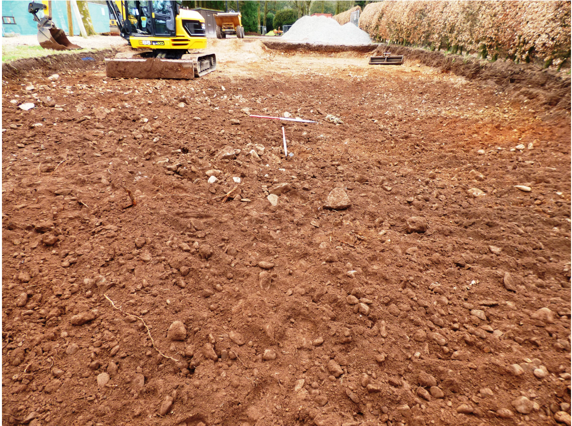
Figure 6b - general post-ex of eastern half (from E)
