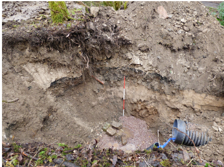
Figure 6b – manhole 1 at SE end (s-facing section) (from S)
