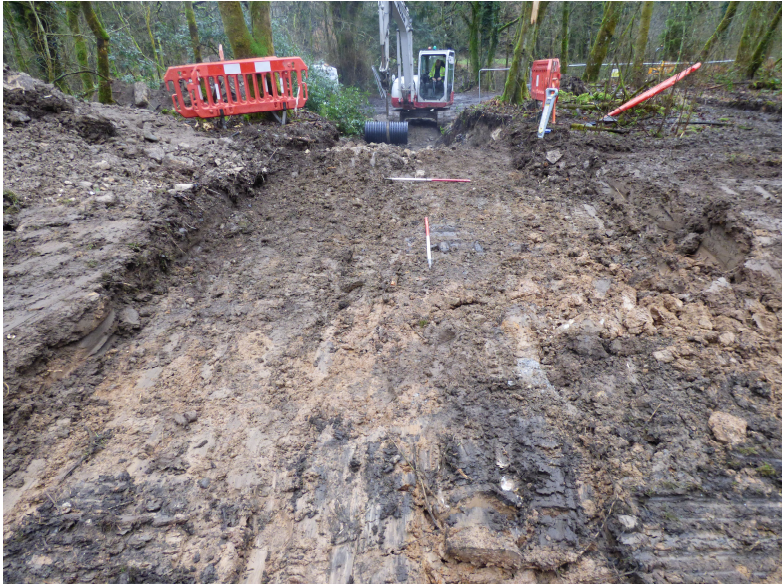
Figure 7a - top of slope after removal of topsoil (from NNW)
