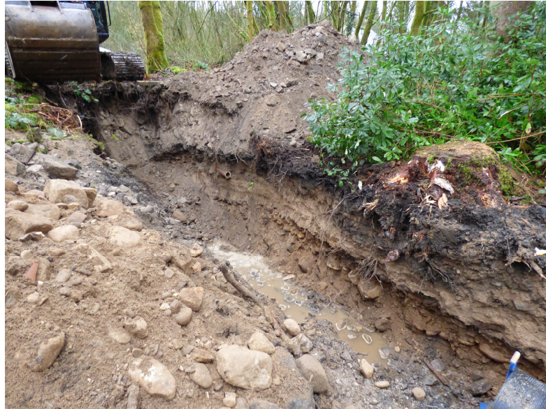
Figure 6a - SE end of monitored section (from S)
