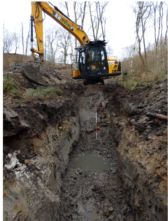
Figure 9d - NNW end of outfall pipe and manhole 2 (from SE)
