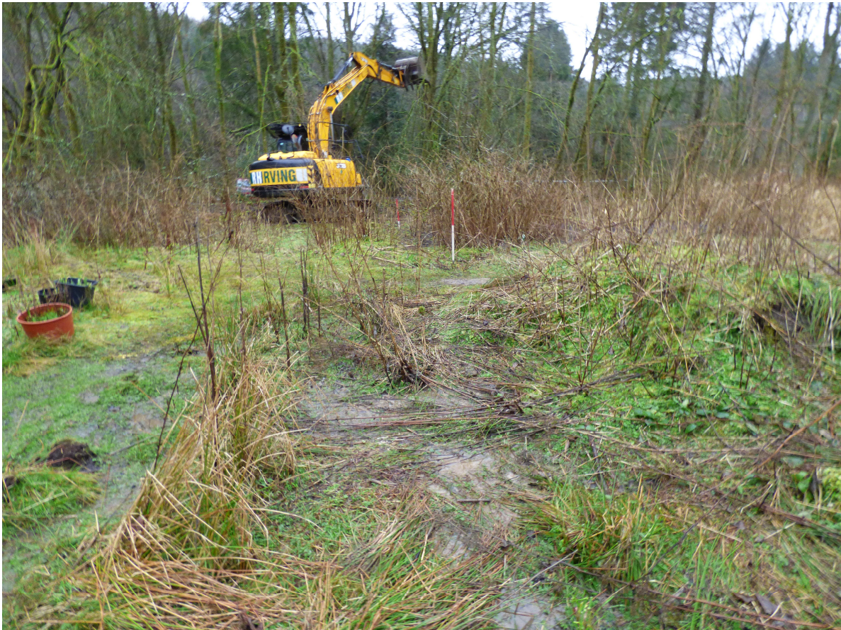
Figure 5c - general pre-ex image - SE end (from NNW)
