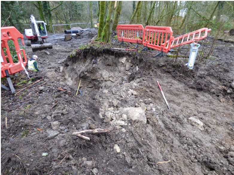
Figure 7c - remains of wall (I) in-situ (from NNE)
