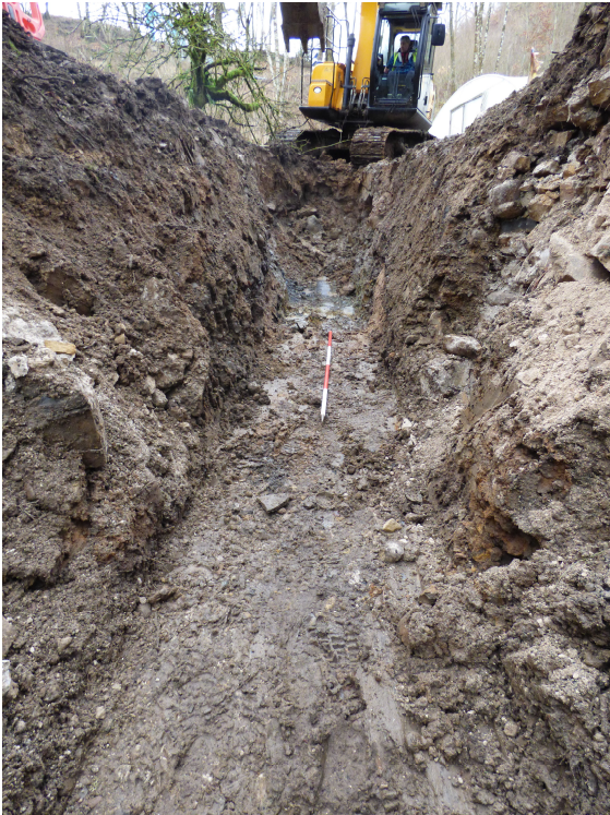
Figure 9a - general of central section of outfall pipe (I) (from SE)
