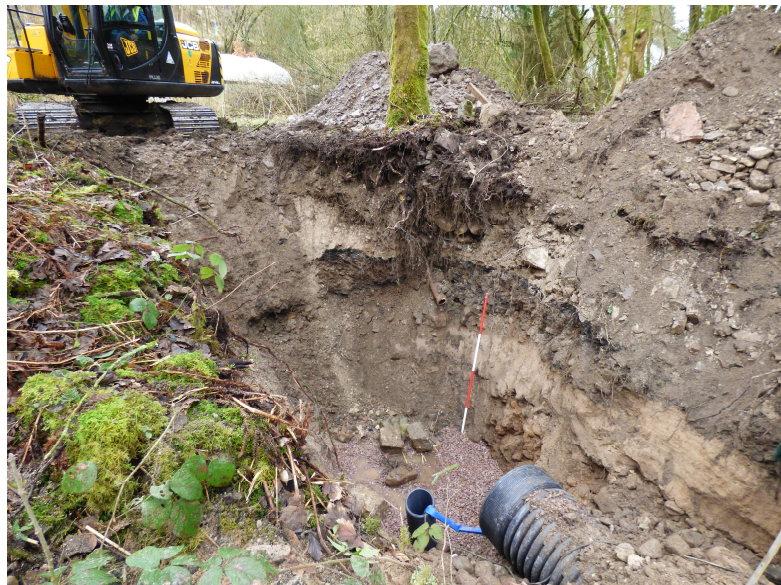
Figure 6c - general of manhole 1 (from SSW)
