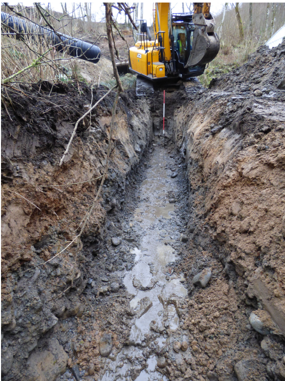
Figure 9c - general of central section of outfall pipe (I) (from SE)
