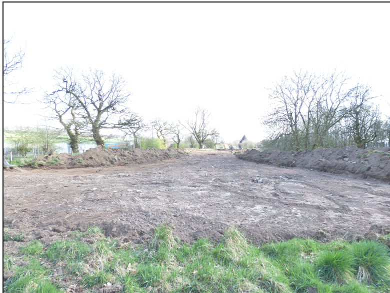
Figure 6b – general post-ex image (from NNW)
