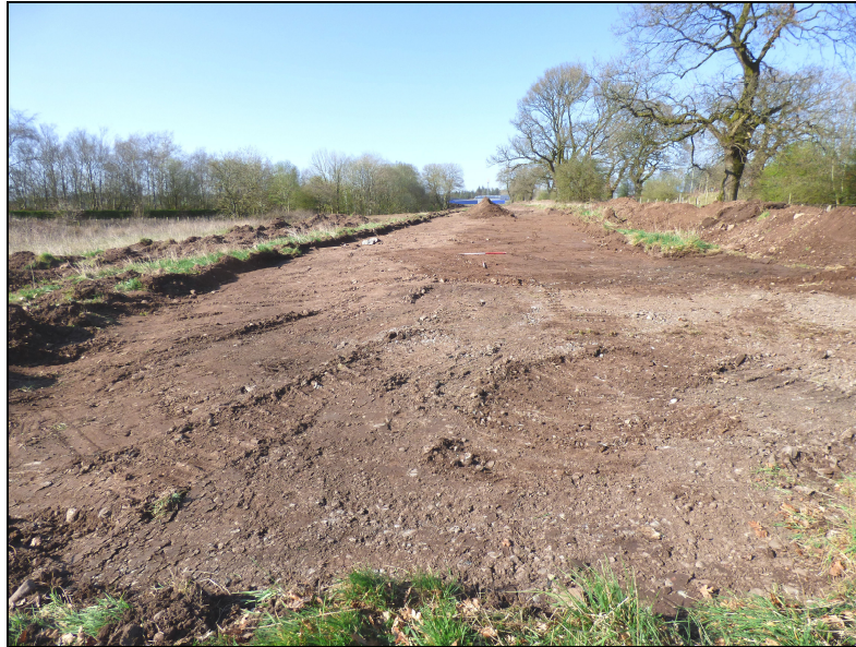
Figure 7a - general post-ex image at southern end (from SSE )
