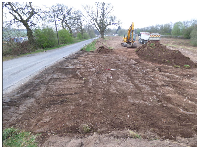
Figure 7c – entrance area (from N)
