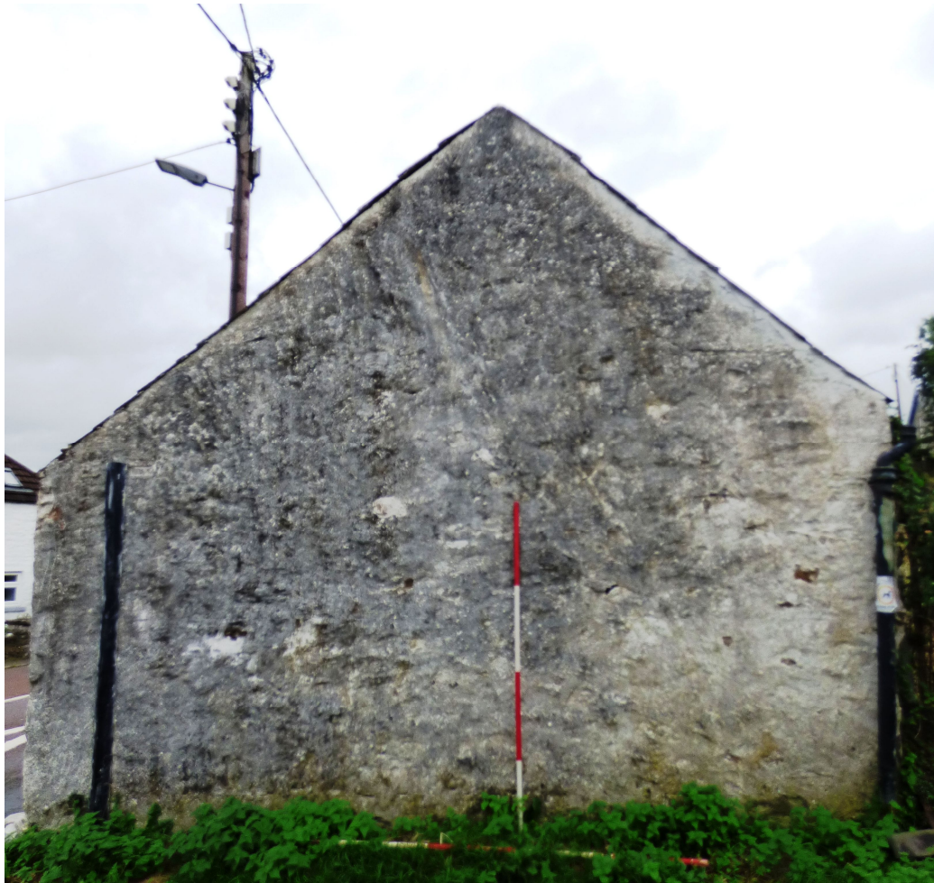
Figure 9a – SSW gable (from SSW)
