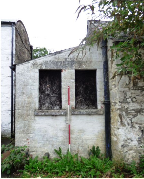
Figure 8a - WNW (front) elevation of brick lean-to (from WNW)
