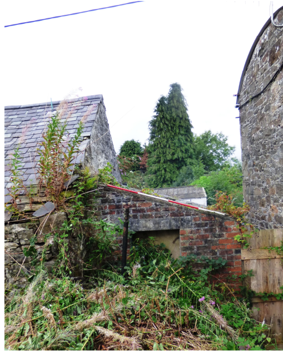
Figure 8b - ESE (rear) elevation of brick lean-to (from ESE)
