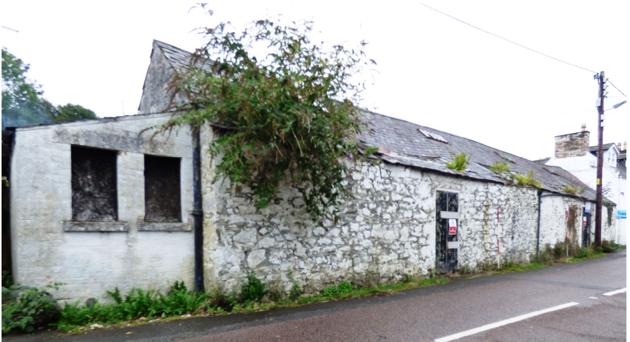
Figure 5a – WNW (front) elevation (from NW)
