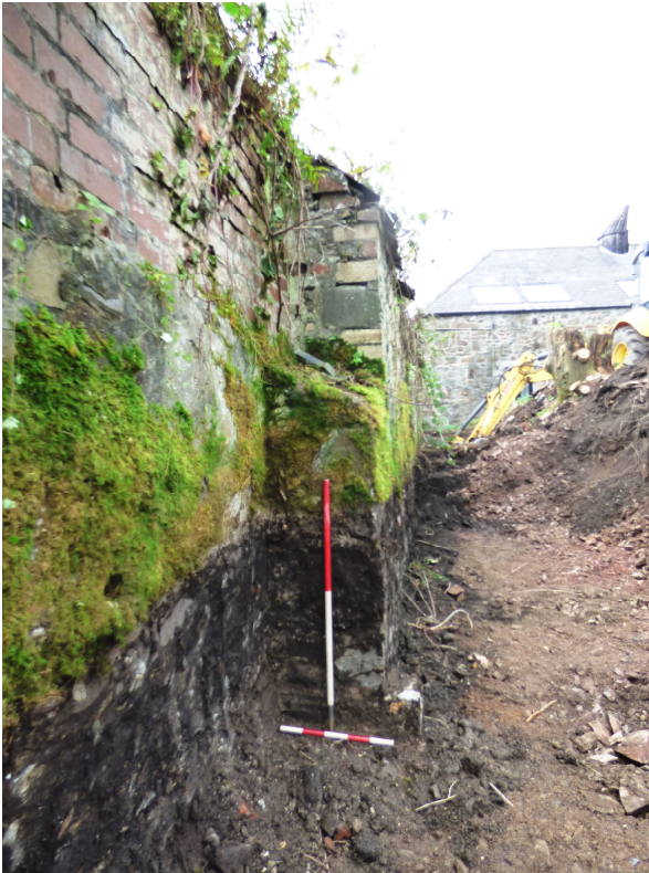
Figure 13a - corner stone / buttress in ESE (rear) elevation (from S)
