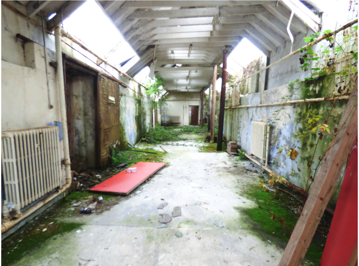
Figure 10b – general of interior from SSW
