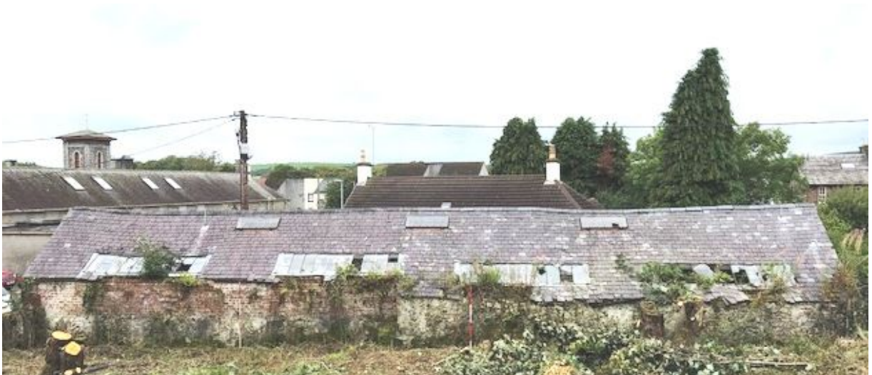
Figure 6b - ESE (rear) elevation (from ESE)
