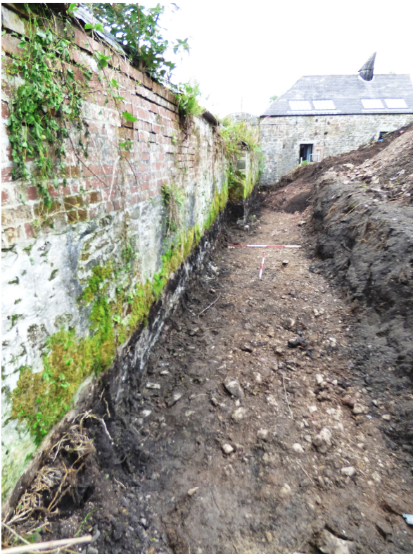
Figure 13c - excavated area adjacent to rear elevation (from SSW)
