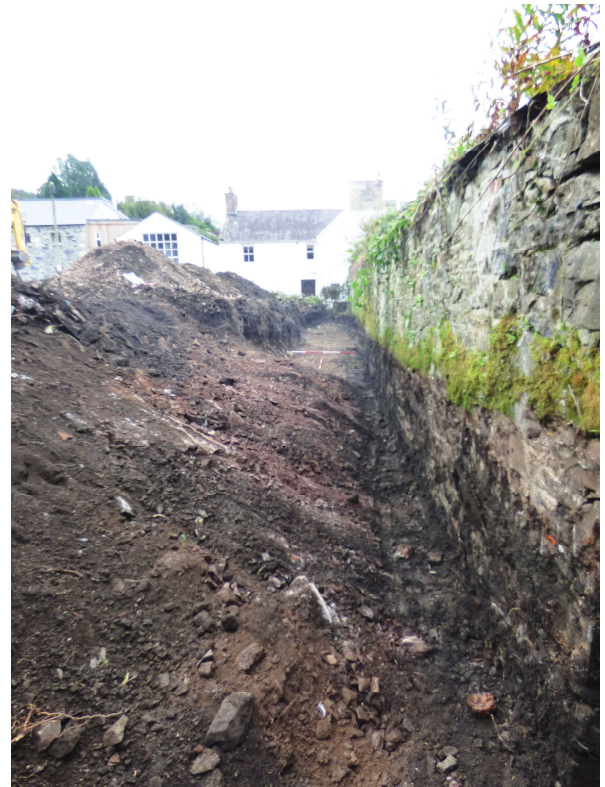
Figure 13d - excavated area adjacent to rear elevation (from NNE)
