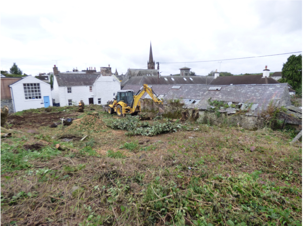
Figure 6a - general of area to the rear (from NE)
