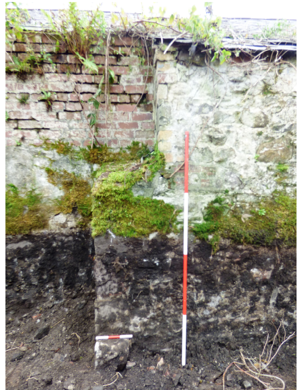
Figure 13b - corner stone / buttress in ESE (rear) elevation (from ESE)
