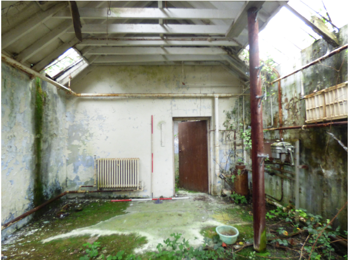
Figure 10a - NNE gable (interior) (from SSW)
