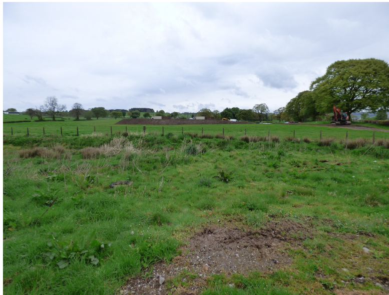
Figure 10a - general pre-ex of shed area (from S)
