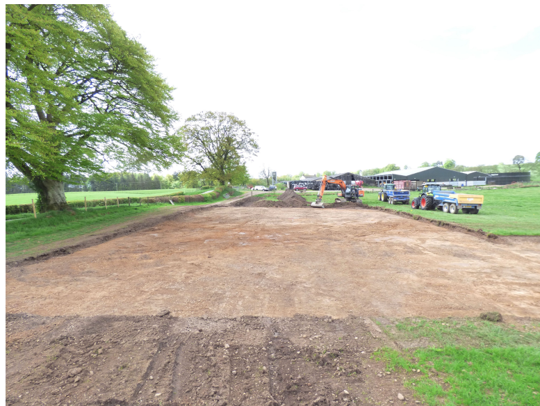
Figure 10b - eastern half during excavation (shed) (from N)
