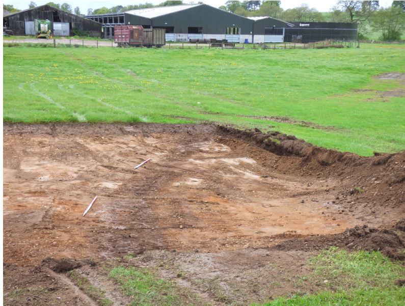
Figure 11a – curved feature / drainage channel (from NE)
