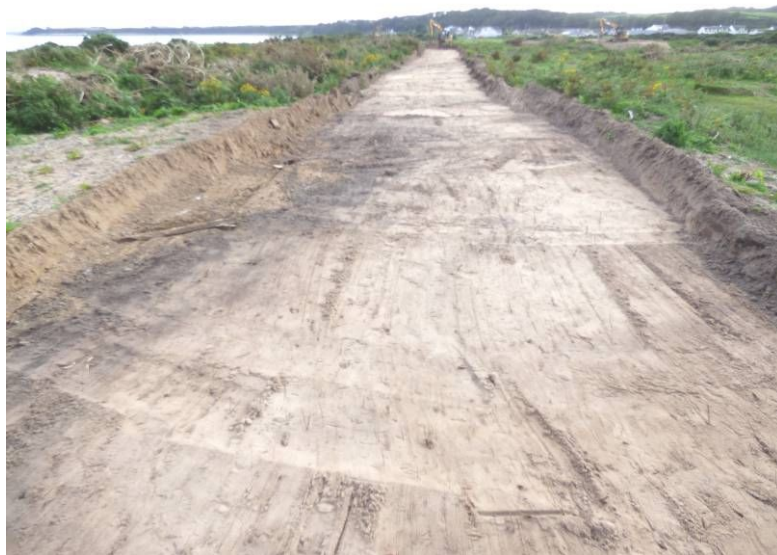
Figure 7b - road section A (from NE)
