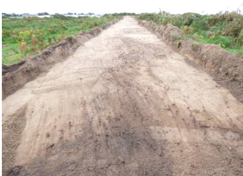
Figure 7a - road section A (from SW)
