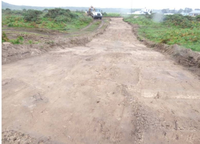
Figure 8a - road section B (from ESE)
