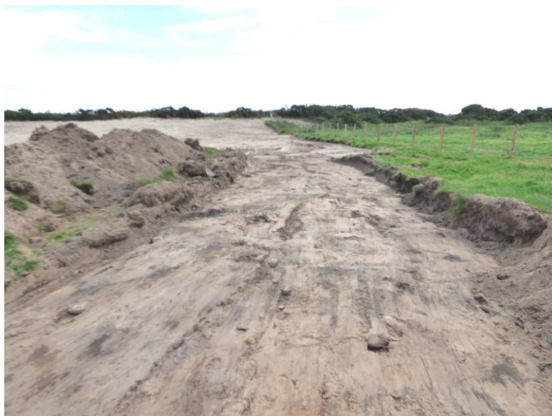
Figure 9c - SSE end of road section (from NNW)
