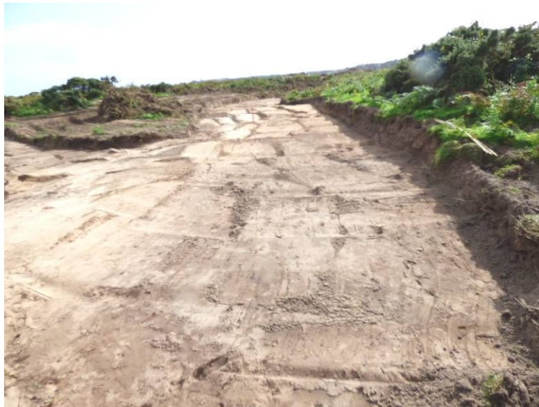
Figure 8b - road section C (I) (from NNE)
