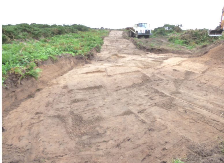
Figure 7c - road section B (from WNW)
