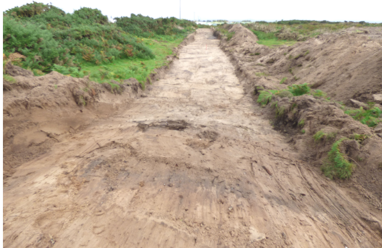
Figure 9a - road section C (IV) (from SSW)
