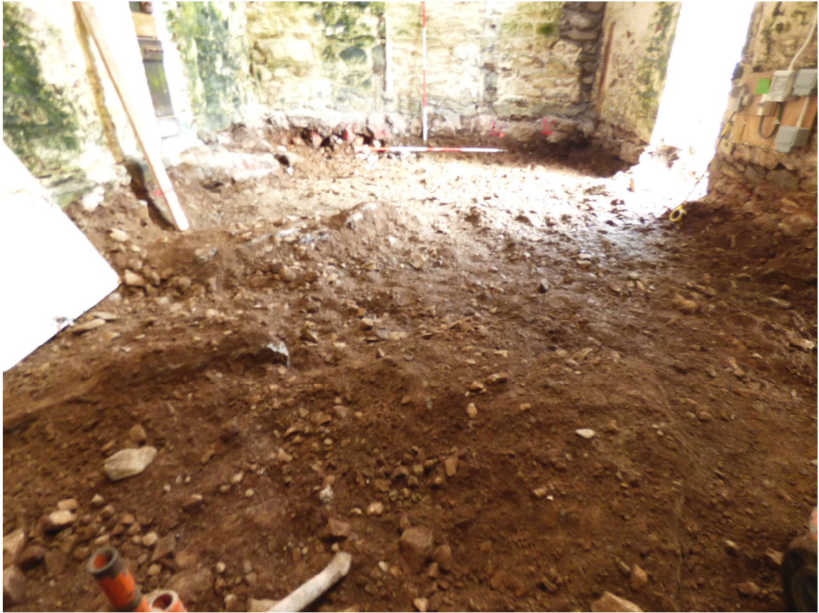
Figure 12a - general after removal of floor within interior (from SW)
