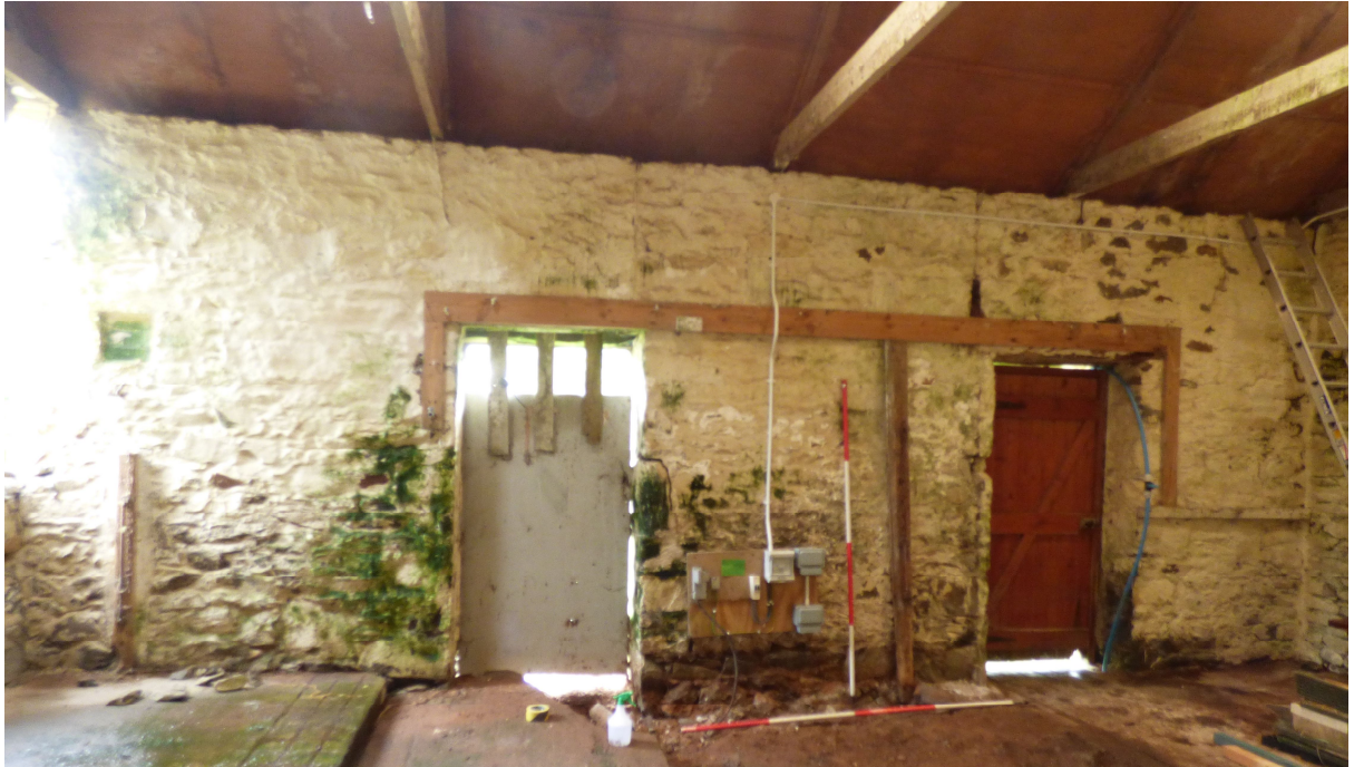
Figure 8a - SE (front) elevation (interior) (from NNW)
