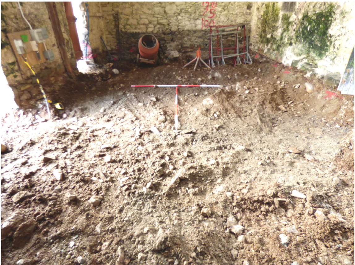
Figure 12b - general after removal of floor within interior (from NE)
