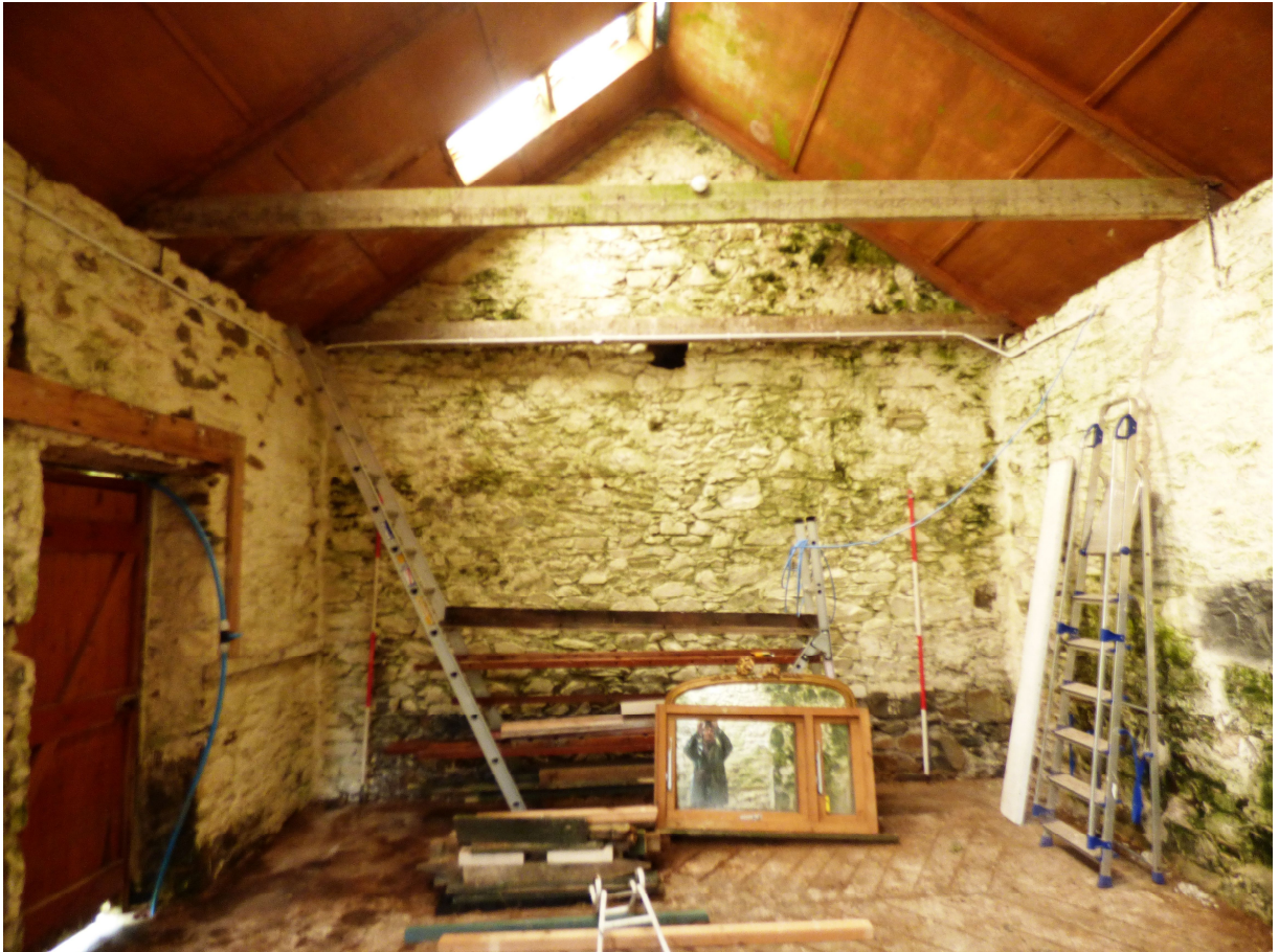
Figure 9a - SW gable (interior) (from NE)
