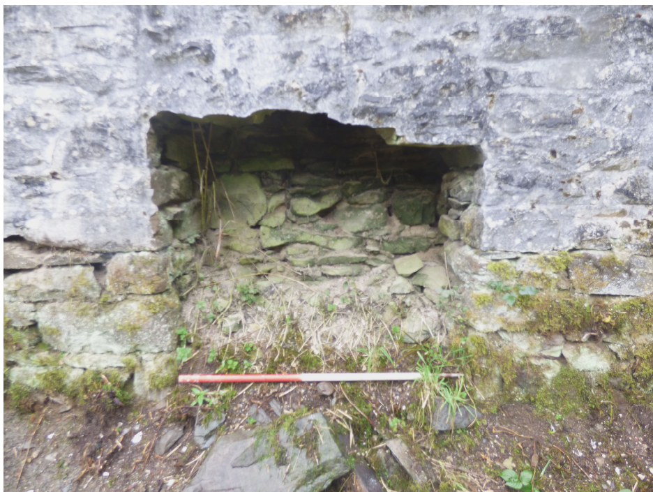
Figure 14b – fireplace within NE gable (from NE)
