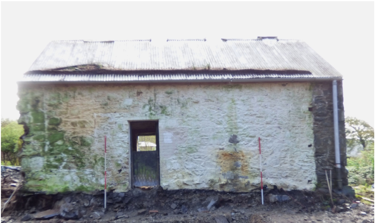
Figure 10b - NW (rear) elevation (from NW) - after removal of shed
