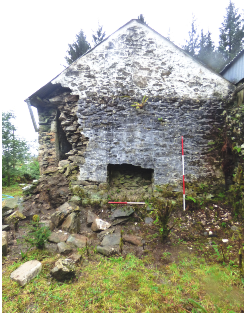
Figure 14a – NE gable (from NE)
