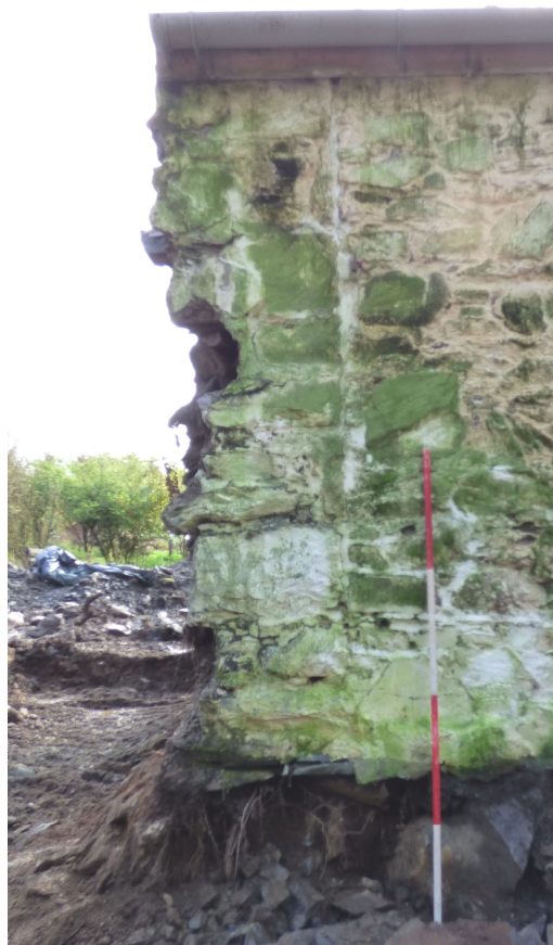
Figure 17b - N corner after removal of partially upstanding wall (from NW)
