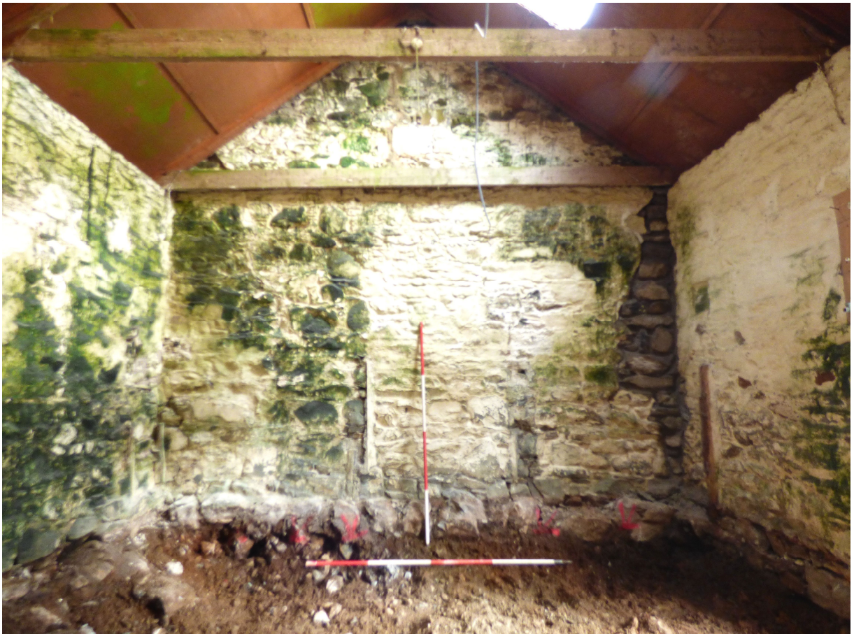
Figure 7b - NE gable (interior) (from SW) - after removal of floor
