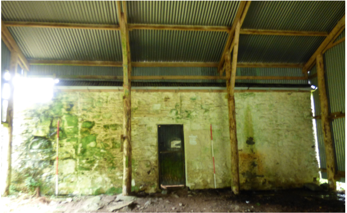
Figure 10a - NW (rear) elevation (from NW)
