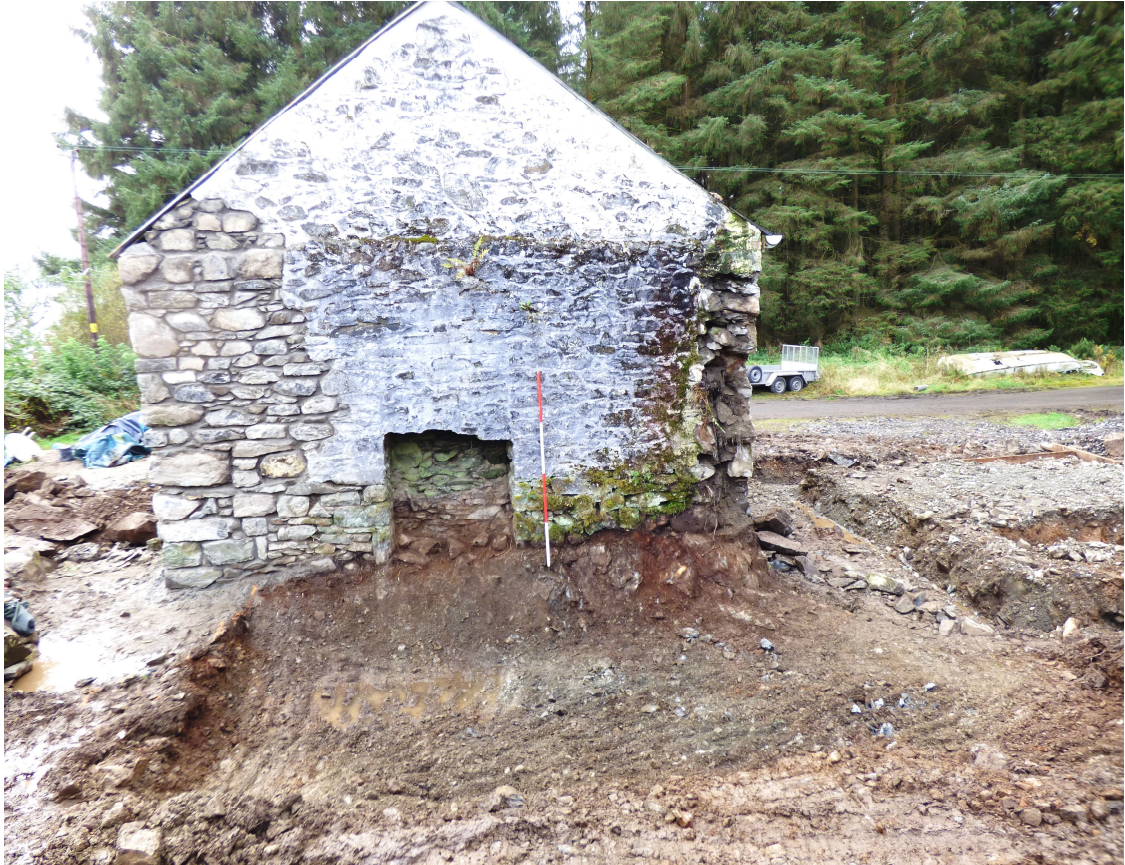
Figure 17a - area of reduced ground for extension to NE (from NE)
