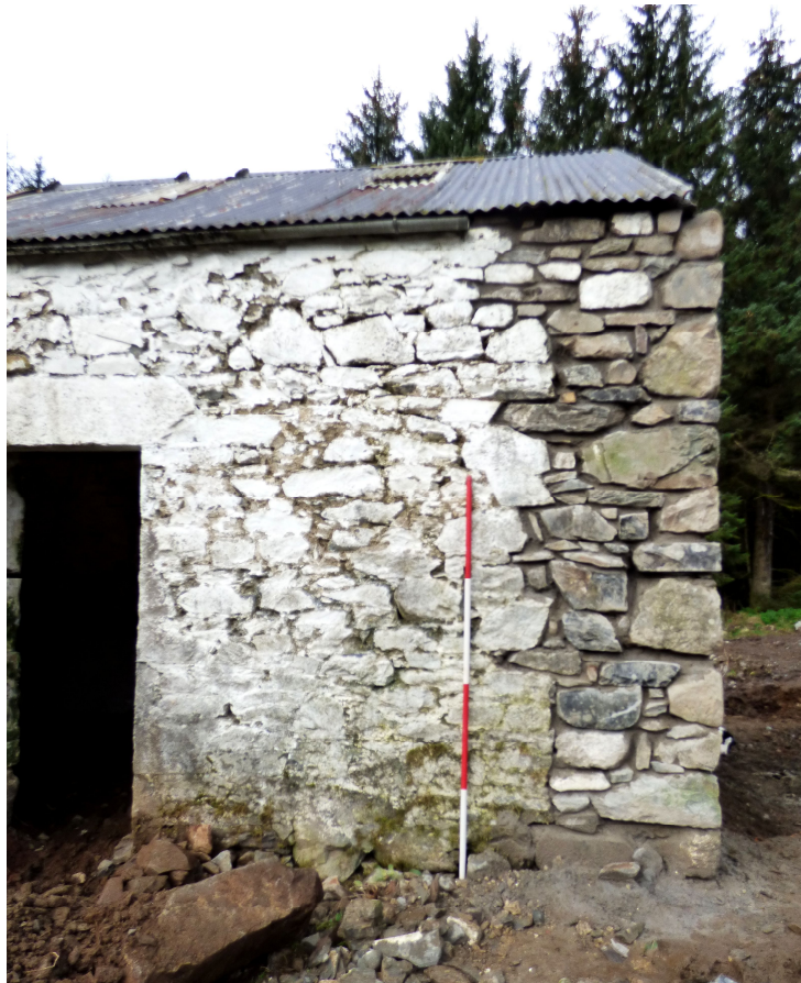
Figure 15c - E corner after repair (from SE)
