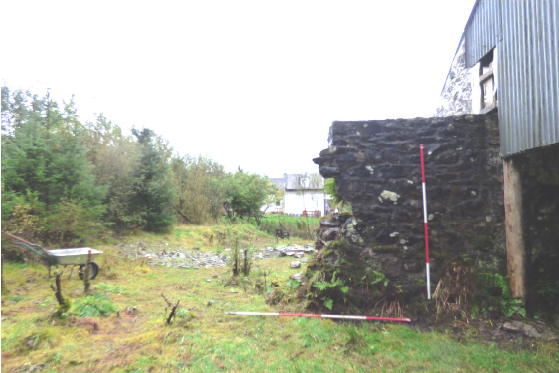
Figure 13a - remains of walling from former structure in NE half (from NW)
