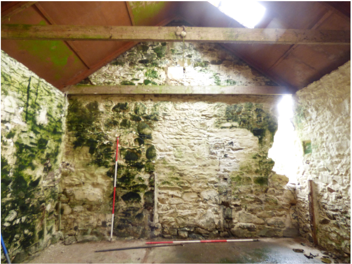
Figure 7a - NE gable (interior) (from SW)
