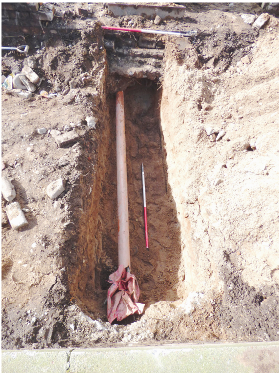
Figure 5c - post-ex of foundation trench A (from ENE)
