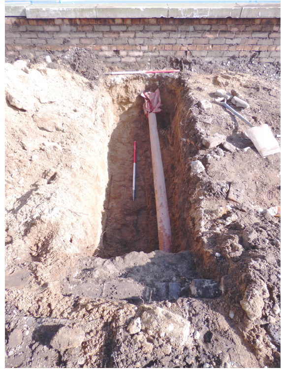
Figure 5b - post-ex of foundation trench A (from WSW)
