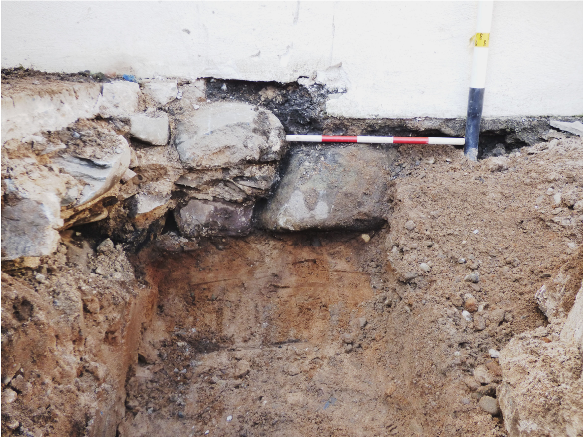
Figure 6a - detail of finds at NNW end of foundation trench B (from SSE)
