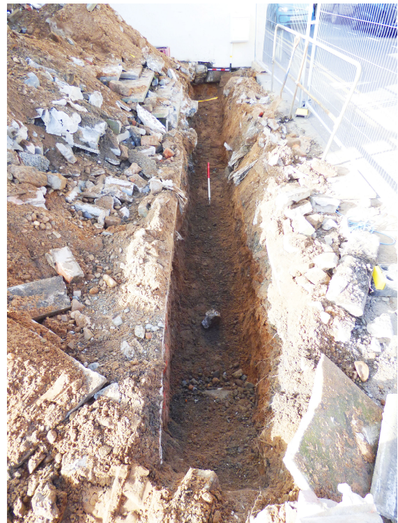
Figure 5d - post-ex of foundation trench B (from SSE)
