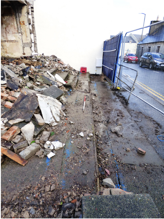
Figure 5a - pre-ex of foundation trench A (from SSE)
