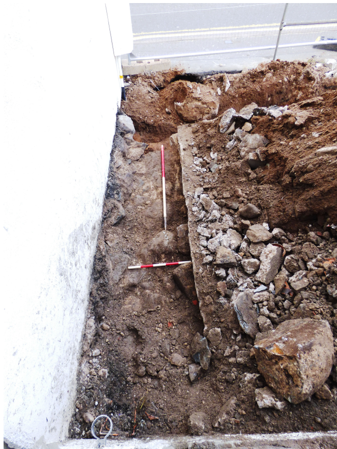
Figure 6b – post-ex of foundation trench C (from ENE)
