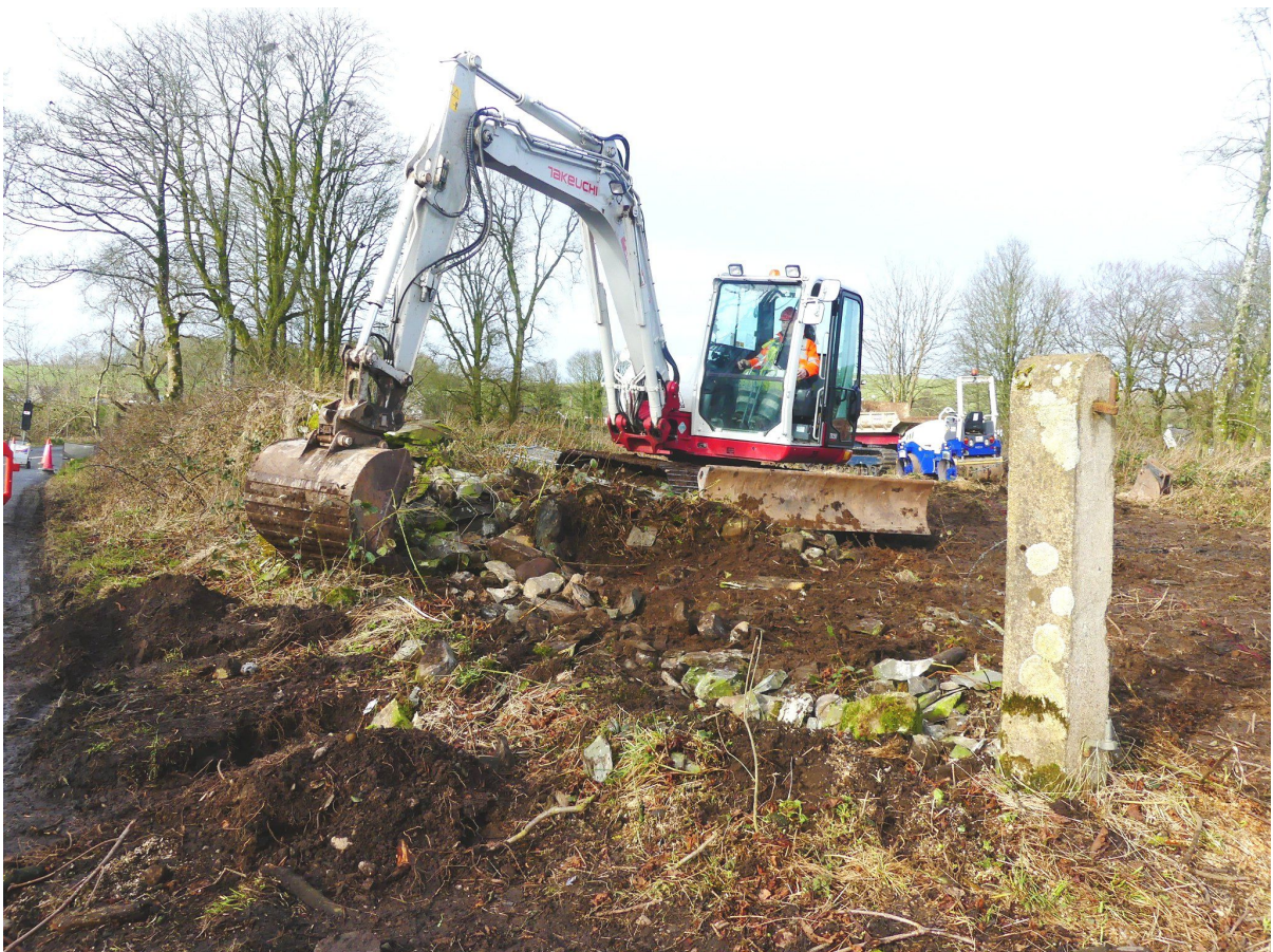
Figure 9b - walling during removal (from E)
