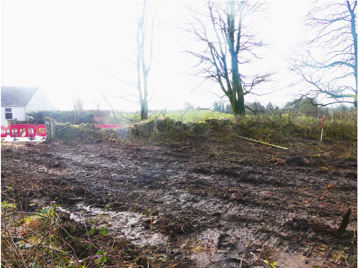
Figure 9a - section of walling to be removed for access (from NNE)
