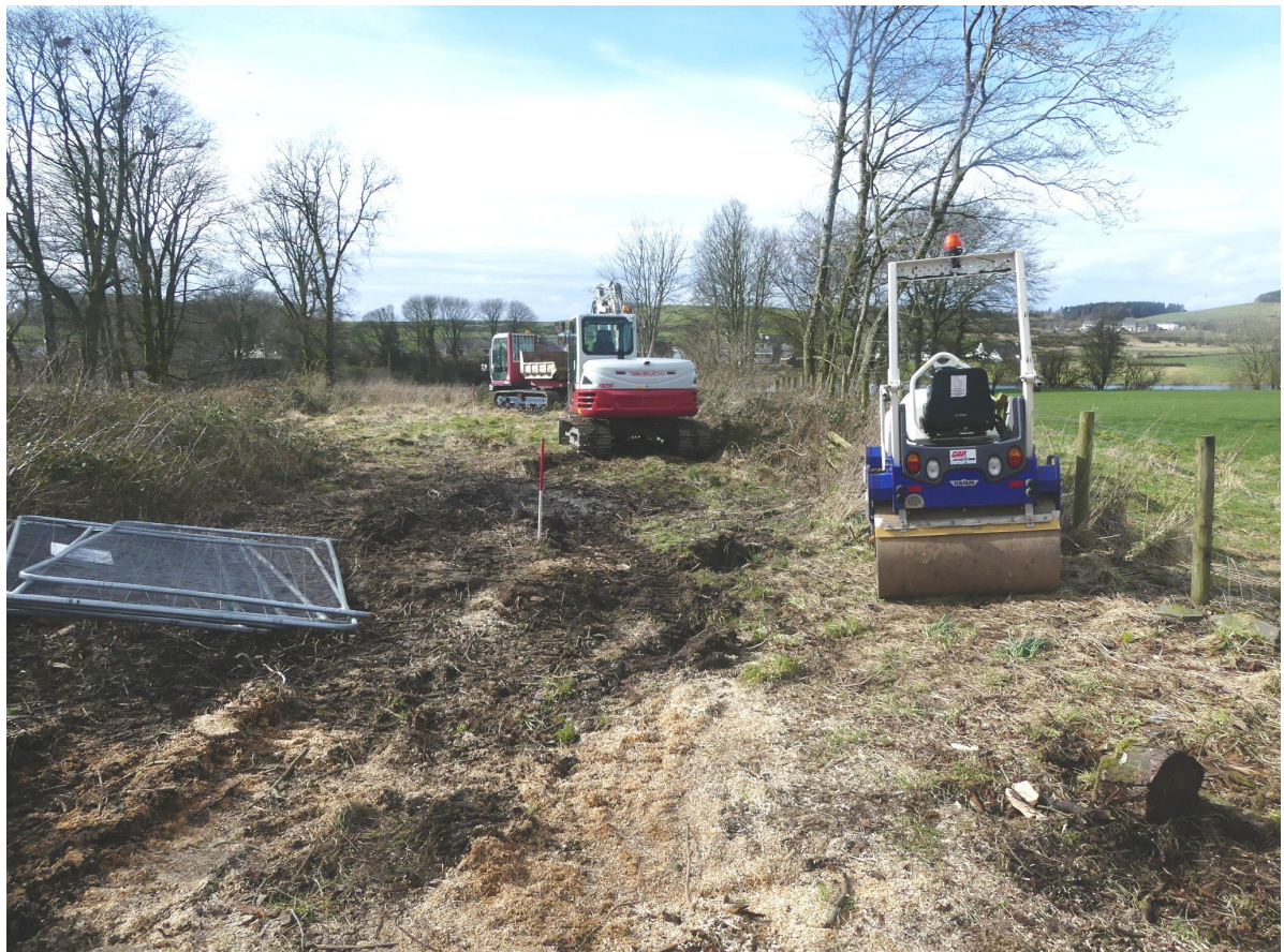
Figure 6b - general pre-ex looking towards barrage (from E)
