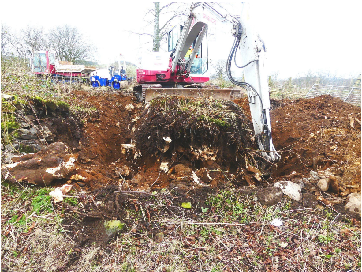
Figure 8b - during removal of stump (III) (from SSW)
