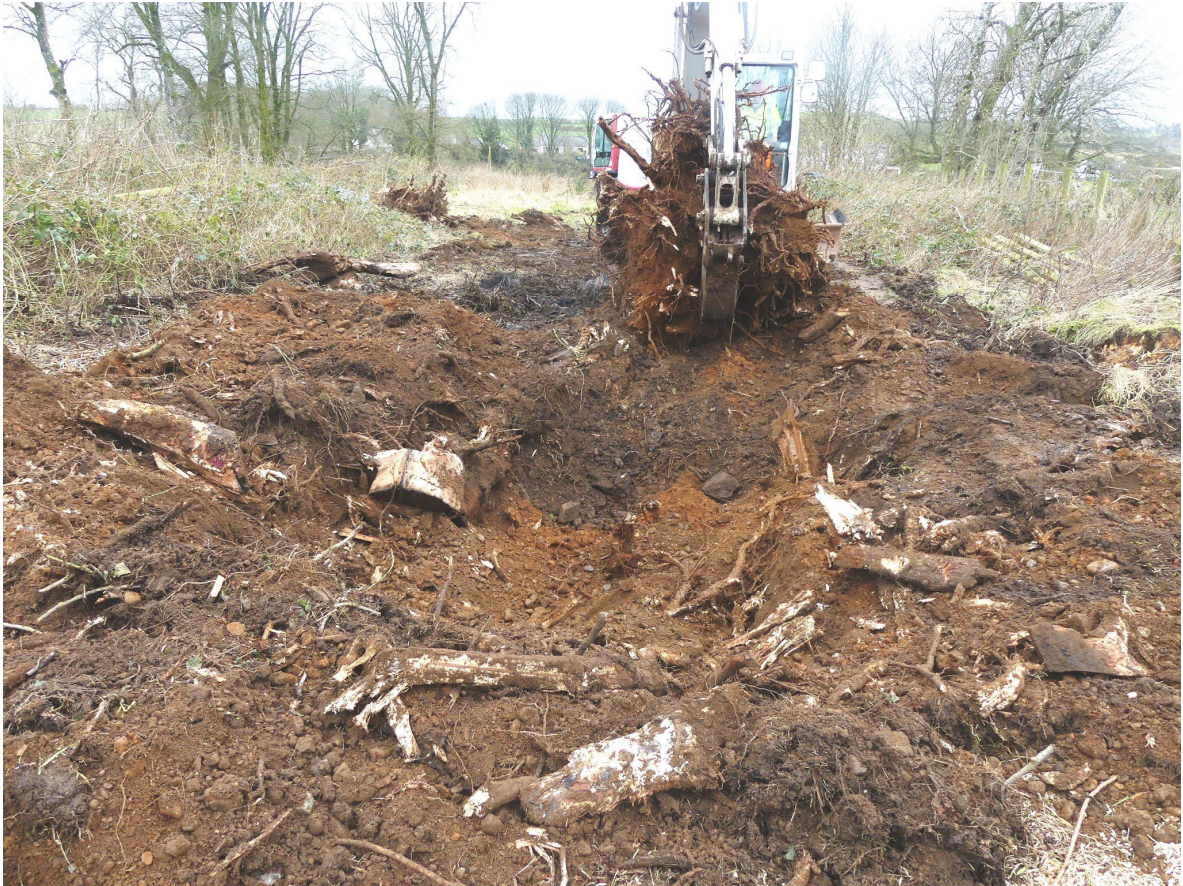
Figure 8a - during removal of tree bowl (II) (from E)
