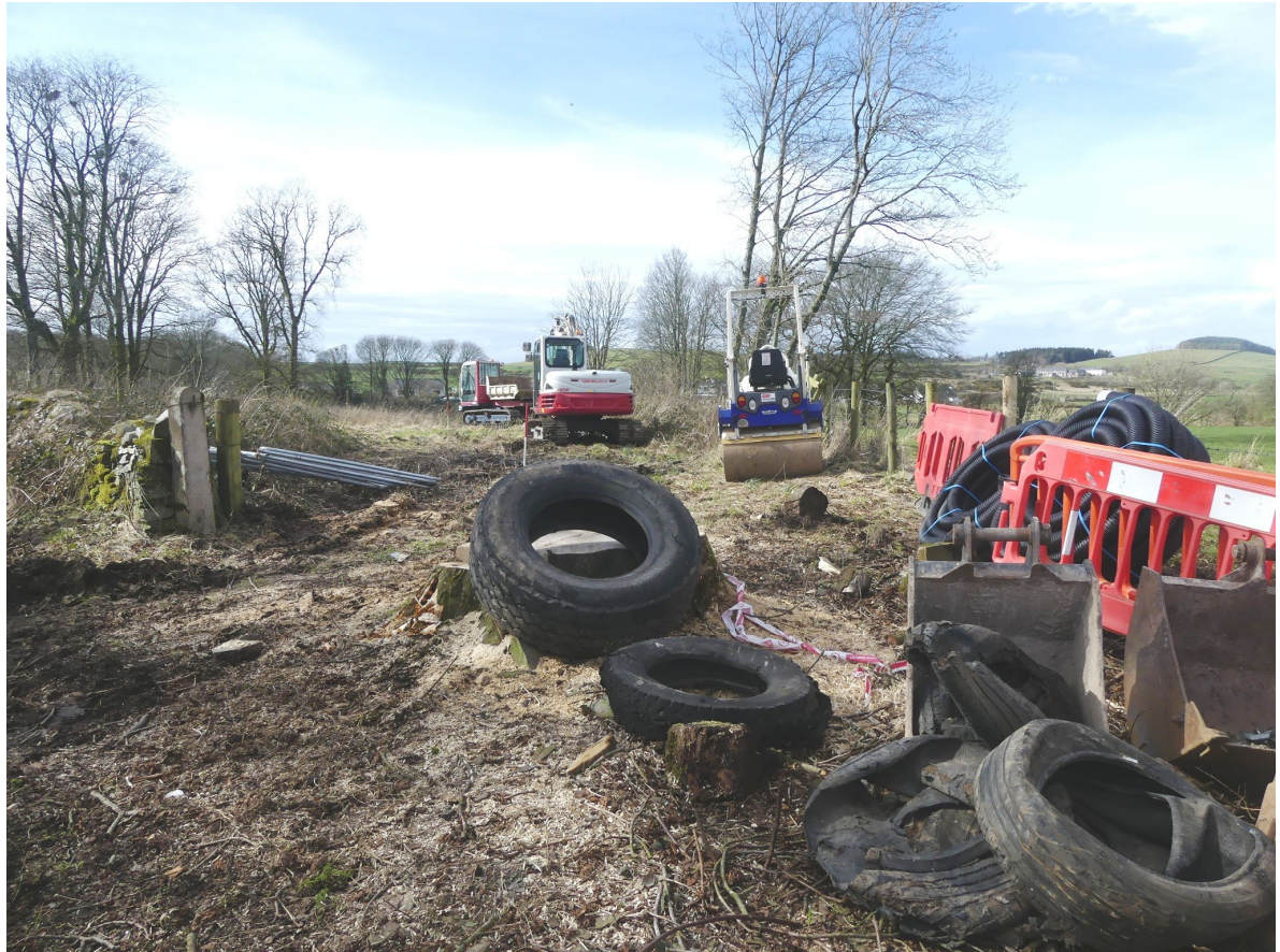
Figure 6a - general pre-ex looking towards barrage (from E)
