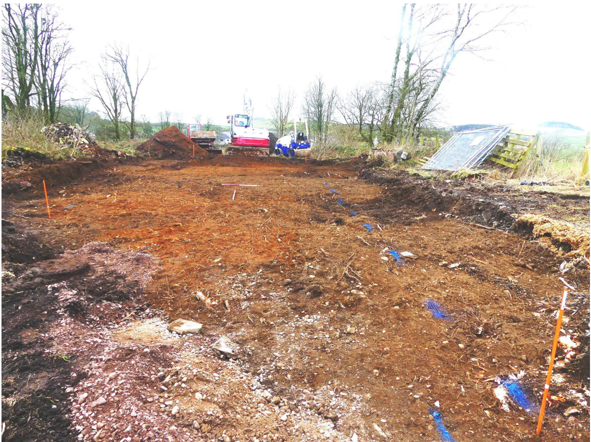
Figure 10b - general post-ex (from E)
