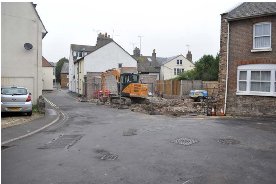
Plate 2: General view of site, looking north.
