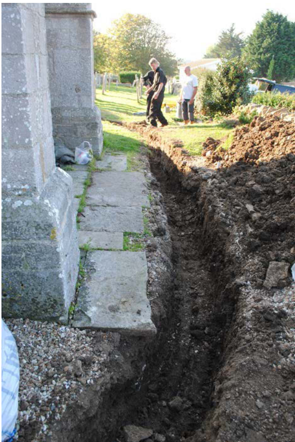
Plate 2: Trenching works west of the West Tower. View from the north.
