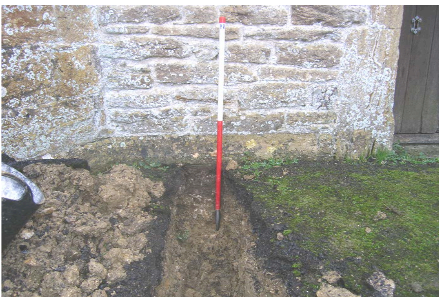
Plate 3: West Tower footings exposed in trench. 1m scale.
