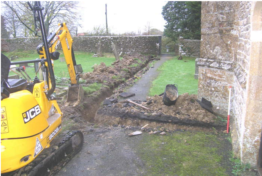
Plate 1: Overview of electricity cable trench, viewed from South. 1m scale.
