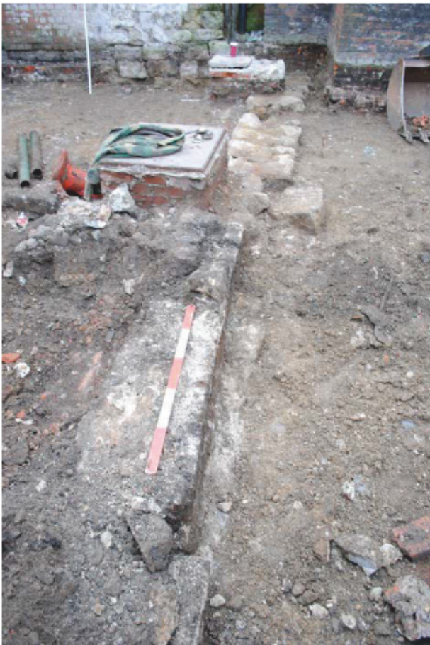
Plate 5: View along Wall 105 showing offset footing beneath. 1m scale.
