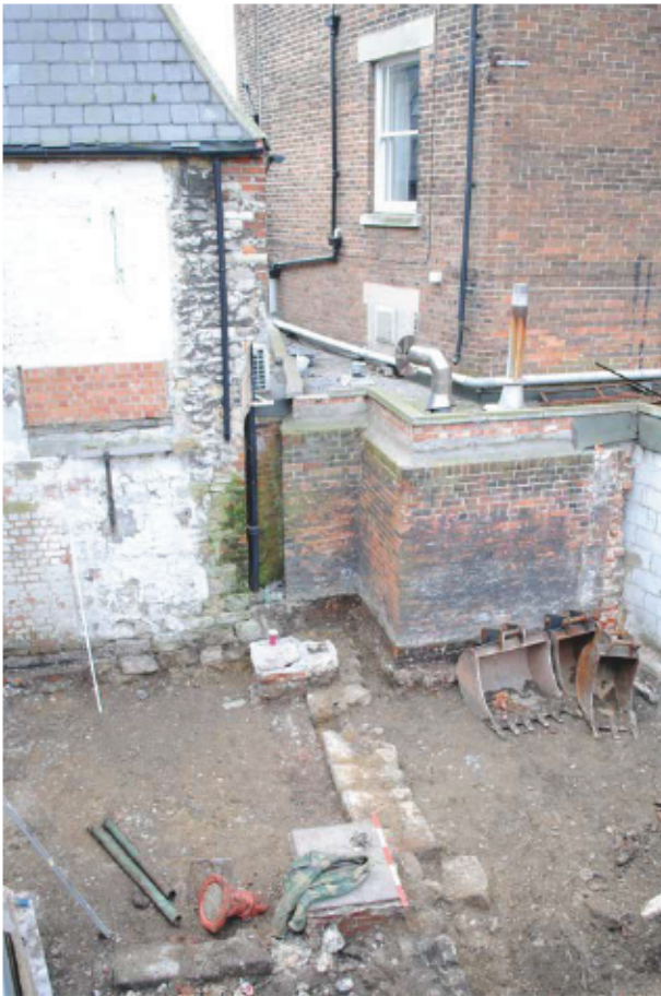
Plate 1: View of southern half of site, with the George Inn behind.
