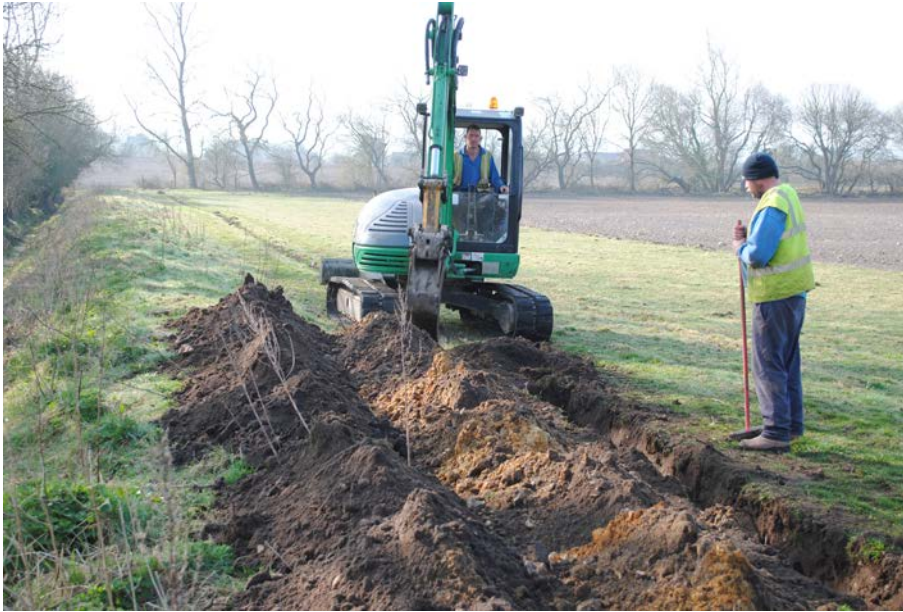
Plate 1: Trenching in the north field, viewed from the north.
