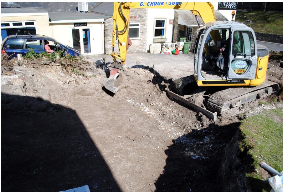
Plate 8: Wall 113 exposed during machining.
