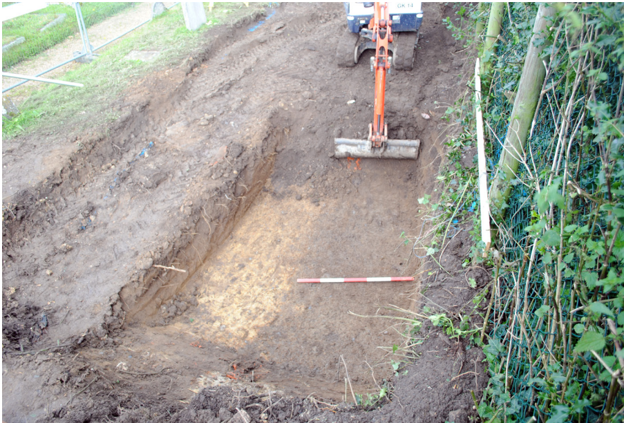
Plate 1: Excavation of footprint of new building showing ditch 101, viewed from south.
