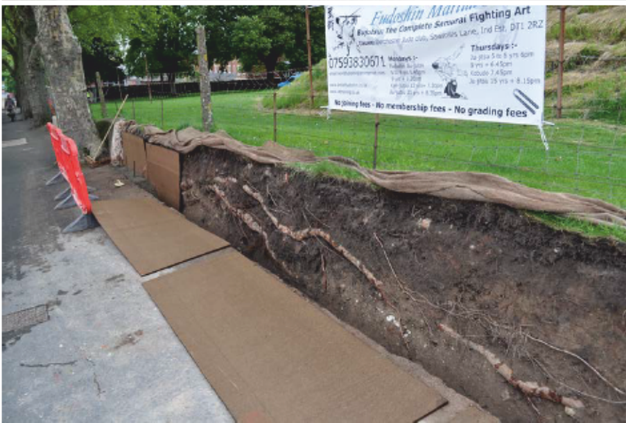
Plate 2: Ditch 102 after removal of retaining wall along Weymouth Avenue.
