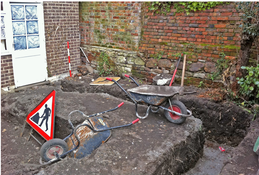
Plate 2: View of footings trench, eastern part, looking Northeast. 1m scale.
