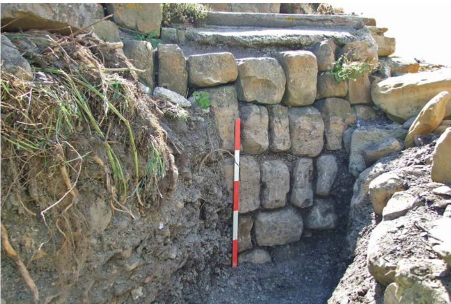
Plate 3: Detail of exposed 17th century quay wall 1004. 1m scale.
