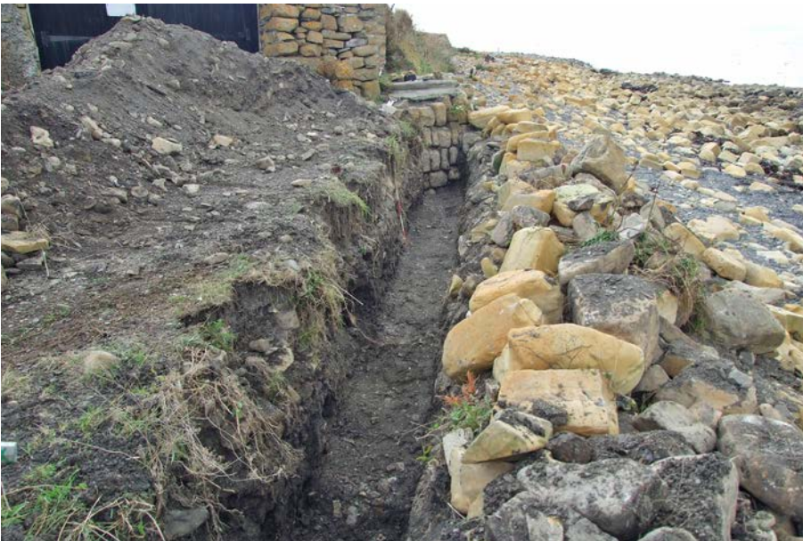
Plate 2: View southwards along construction trench. 1m scale.
