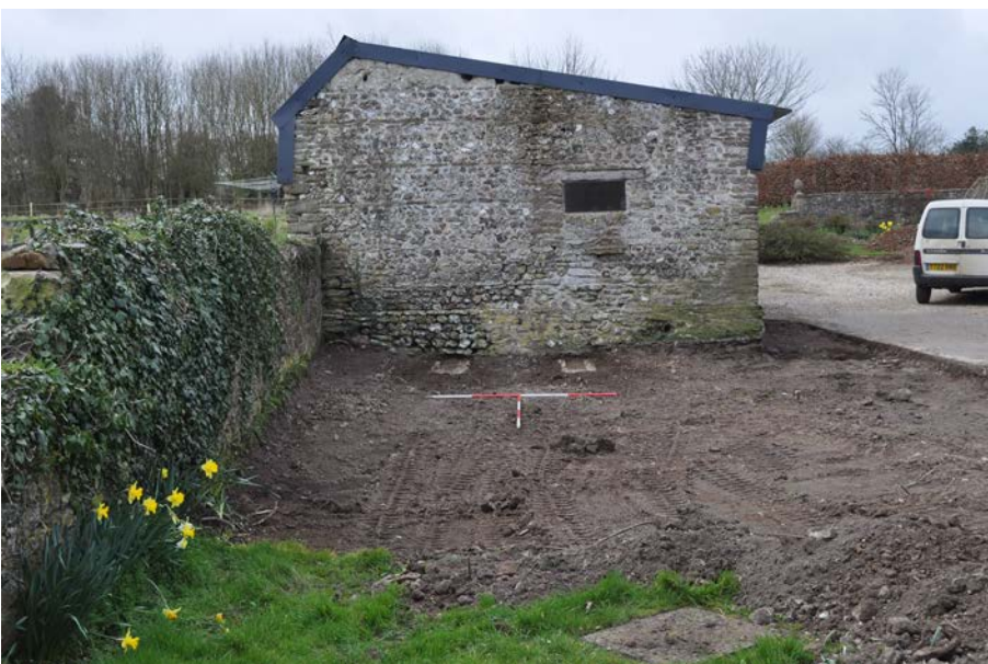
Plate 2: View of new parking area after stripping, looking south west, with concrete base 103 in background. 2m scales.
