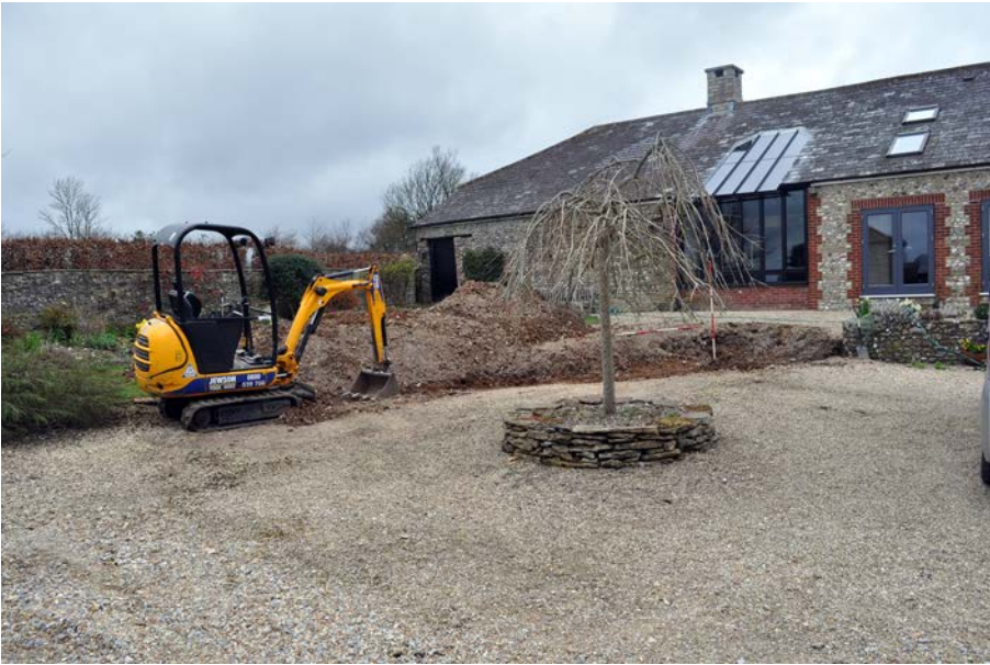
Plate 4: View of new retaining wall trench, looking south west. 2m scales.
