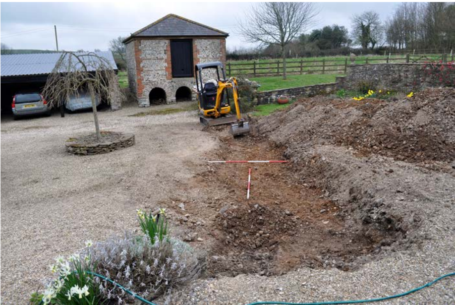
Plate 5: View along line of new retaining wall trench, looking south east. 2m scales.
