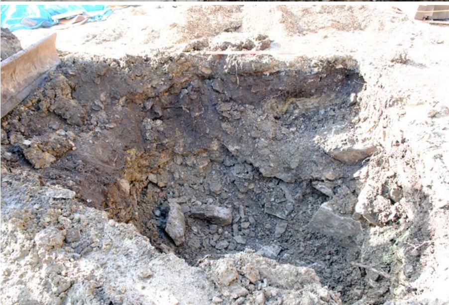
Plate 3: Excavation of soakaway pit 1 in progress. View from north.
