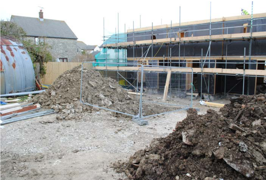
Plate 2: Overview of development. View from south west.
