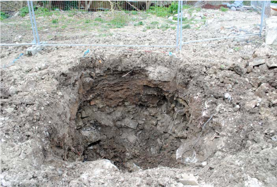
Plate 5: Soakaway pit 3, viewed from east. 1m scale.
