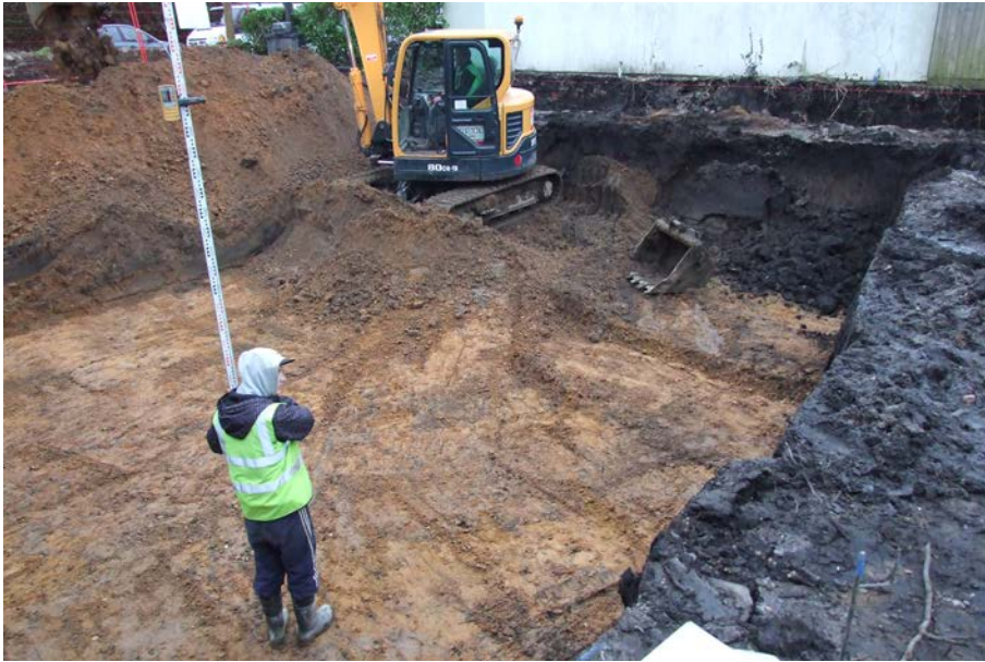
Plate 7: Mechanical clearance of natural deposits within basement area. View from SSE.
