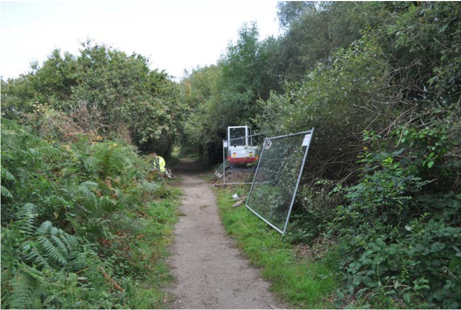
Plate 1: View of location of drain trench from south.
