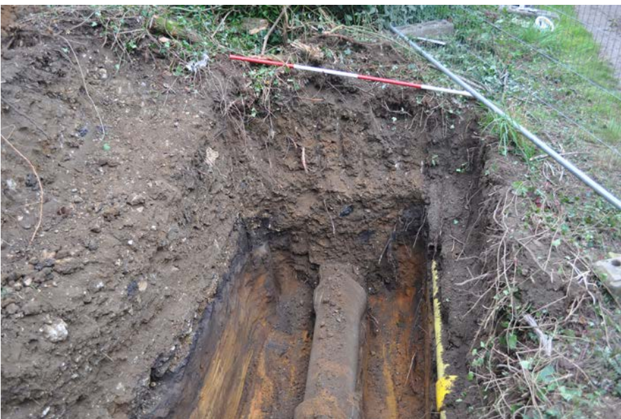
Plate 3: Drain repair trench viewed from north. 2 m scale.
