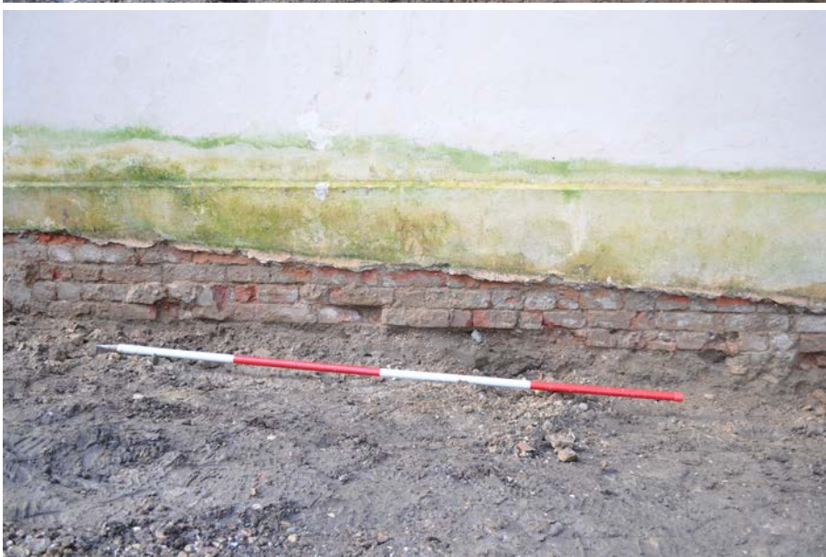
Plate 3: Detail of brick plinth of original cottage east wall. 2m scale.
