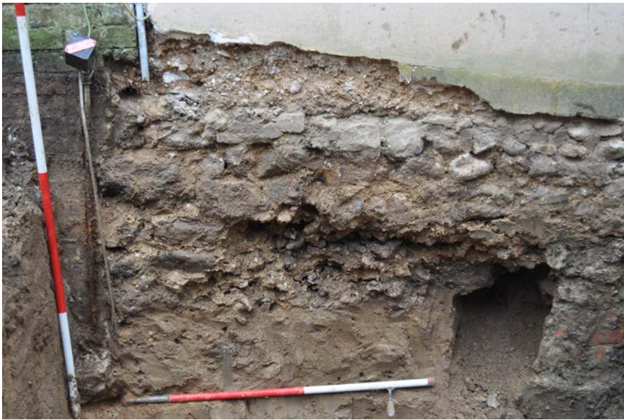
Plate 7: Footings 105 at south end of cottage and junction with the south extension in underpinning pit 13/14. 2m & 1m scales.
