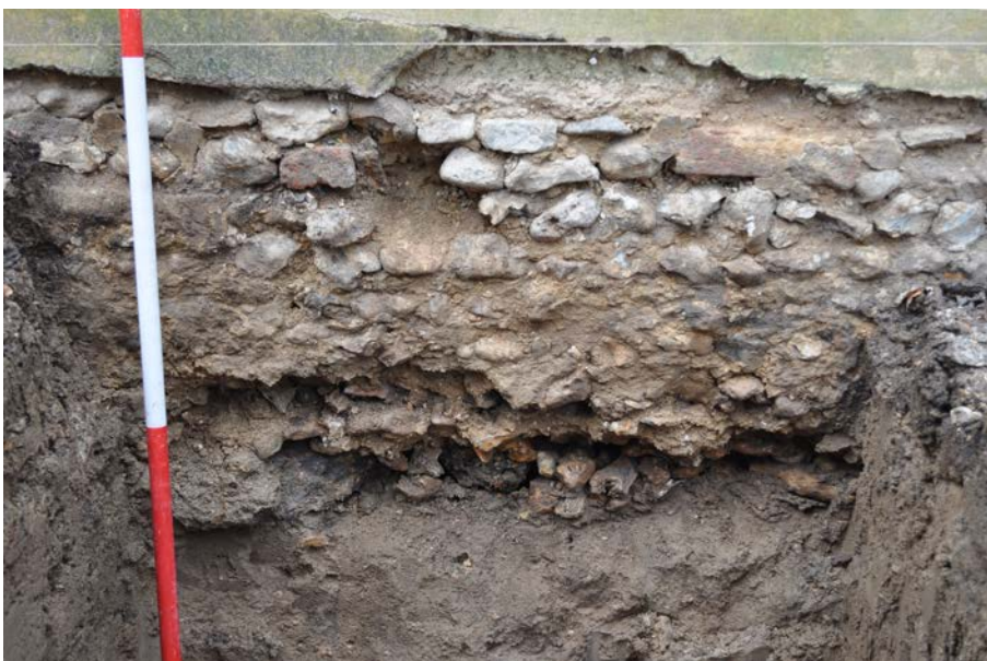
Plate 6: Detail of flint footings 105 in underpinning pit 12.
