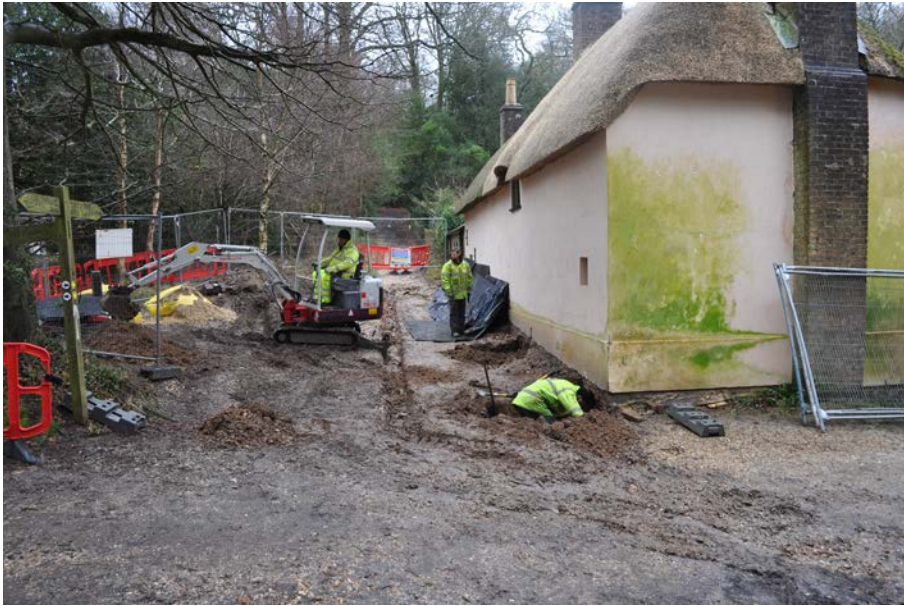
Plate 1: General view of site during underpinning works, looking south.
