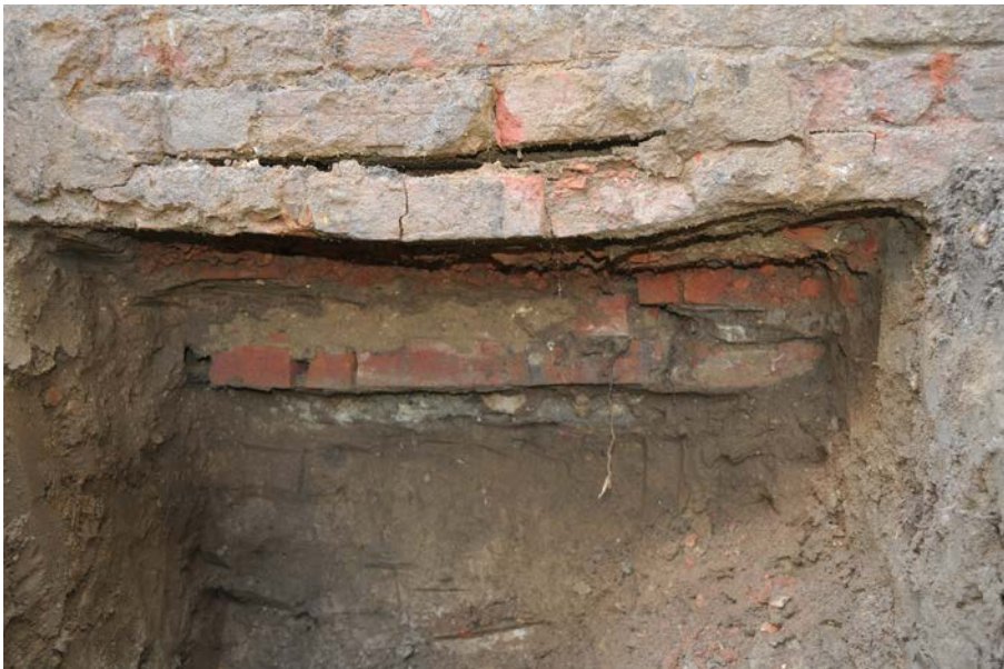
Plate 5: Detail beneath brick plinth 103 in underpinning pit 7, showing relationship with floor.
