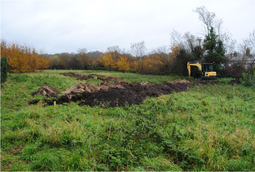
Plate 1: Overview of trenches looking ESE from Knighton Lane.
