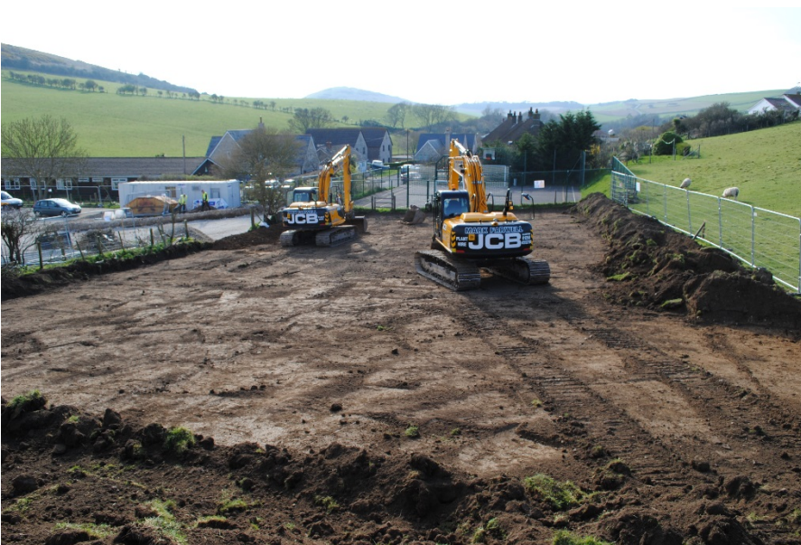
Plate 8: Temporary works compound after topsoil stripping. View from east.
