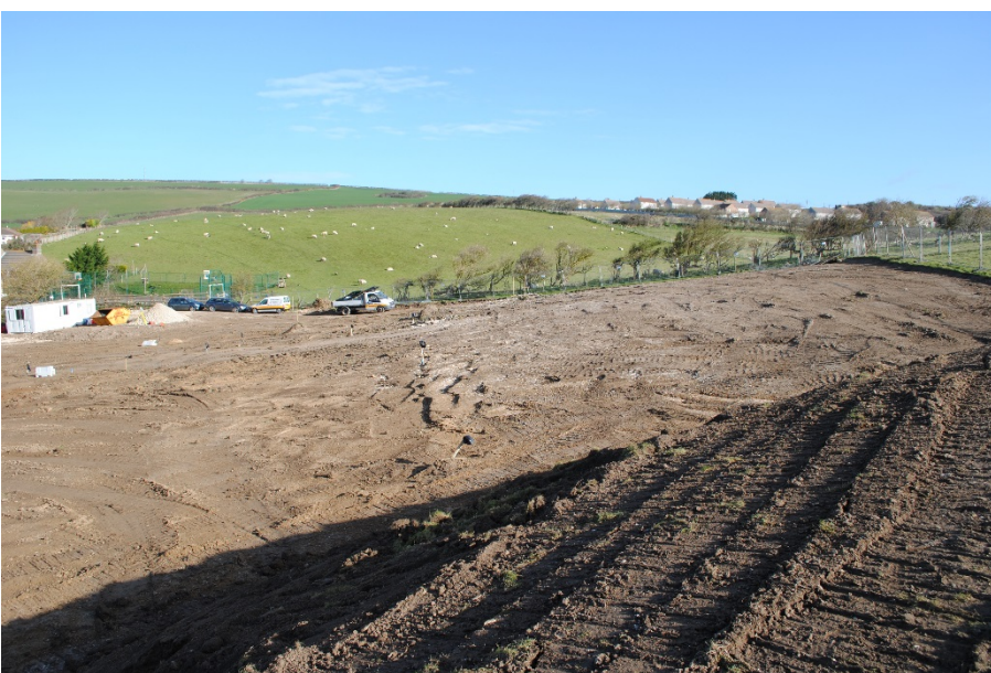
Plate 3: Eastern area of site after topsoil stripping. View from south.
