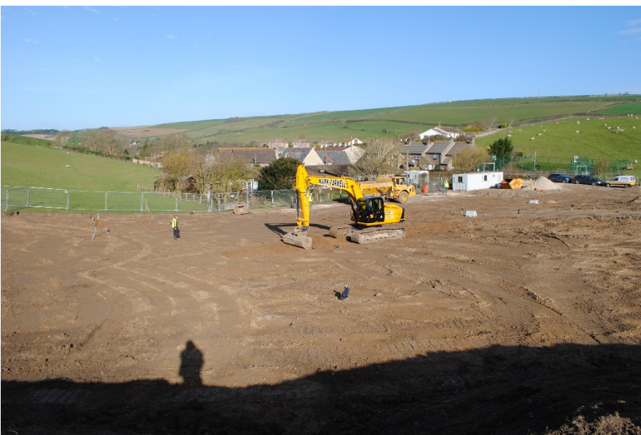
Plate 2: Central area of site after topsoil stripping. View from south east.
