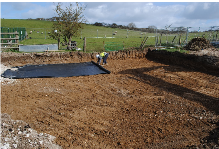
Plate 5: 'Turning circle' area after secondary ground reduction. View from south west.
