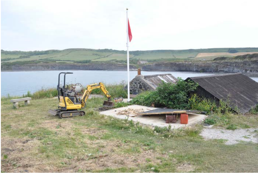
Plate 1: View of site before groundworks, viewed from south east.
