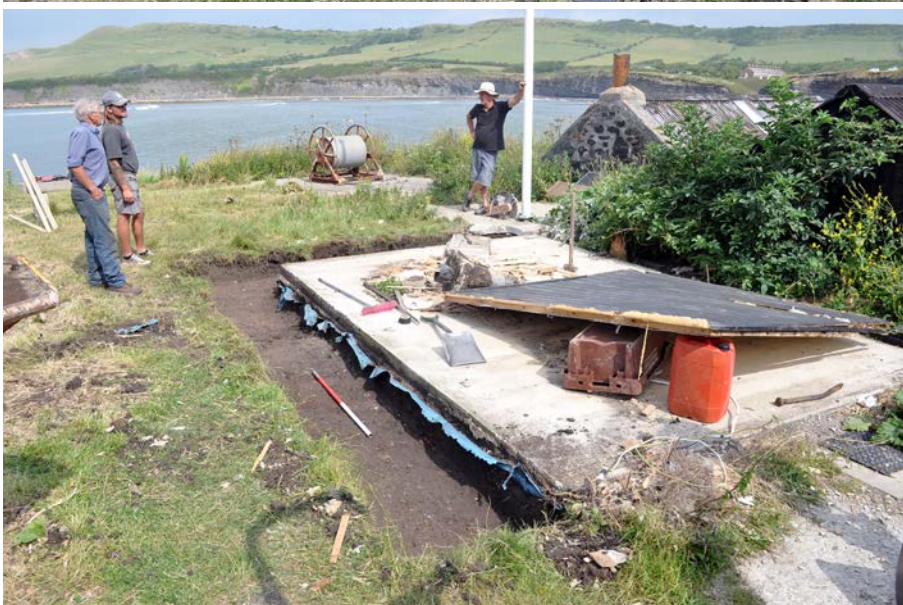
Plate 3: South side of concrete base after excavation, viewed from ESE. 1m scale.
