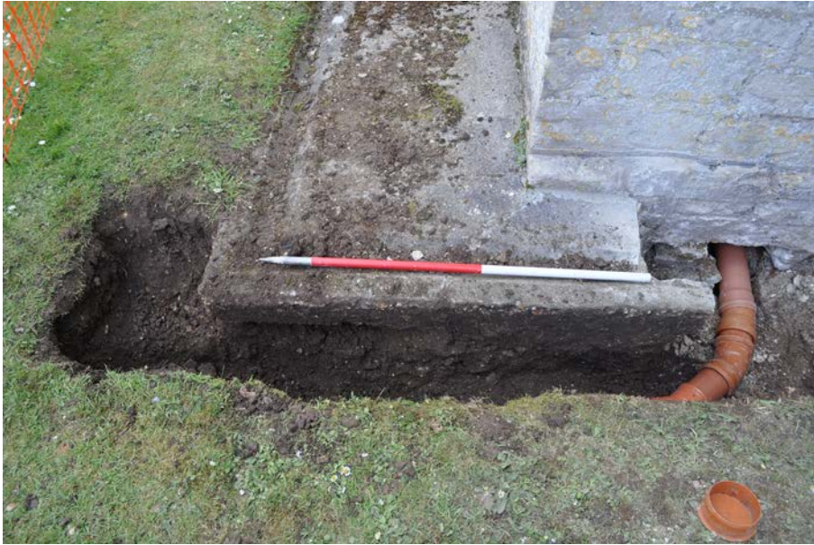
Plate 4: Foul drain through west wall of nave and west end of drain trench. View from west. 1m scale.
