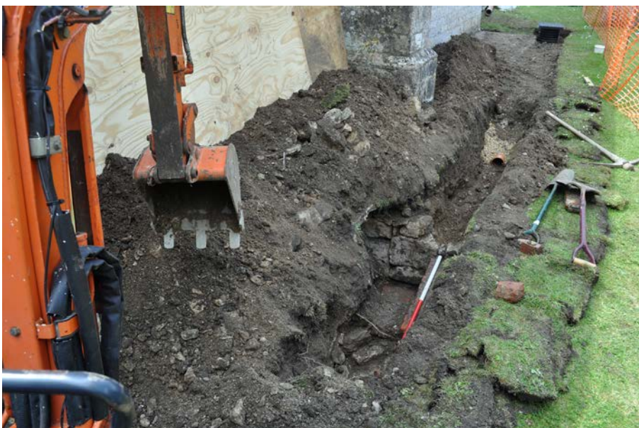
Plate 6: View of vault entrance 126 with 1m scale on steps 122 and revetment wall 124 behind. View from north east.
