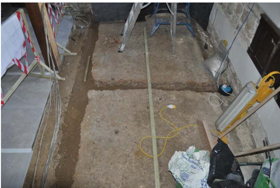
Plate 3: Surface 101 after excavation of conduit channels.
