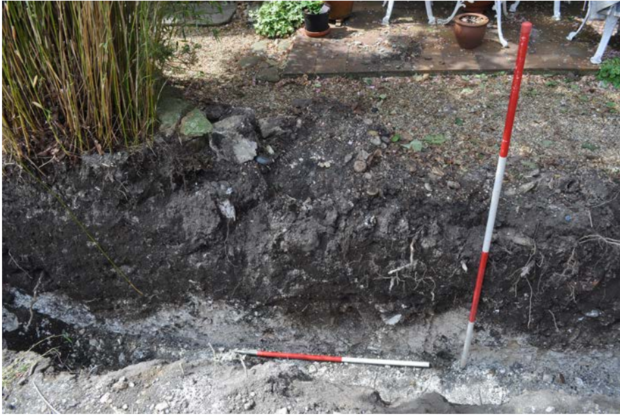
Plate 1: Ditches 103, 105 and 107 along western boundary of the site, viewed from east. 1m & 2m scales.
