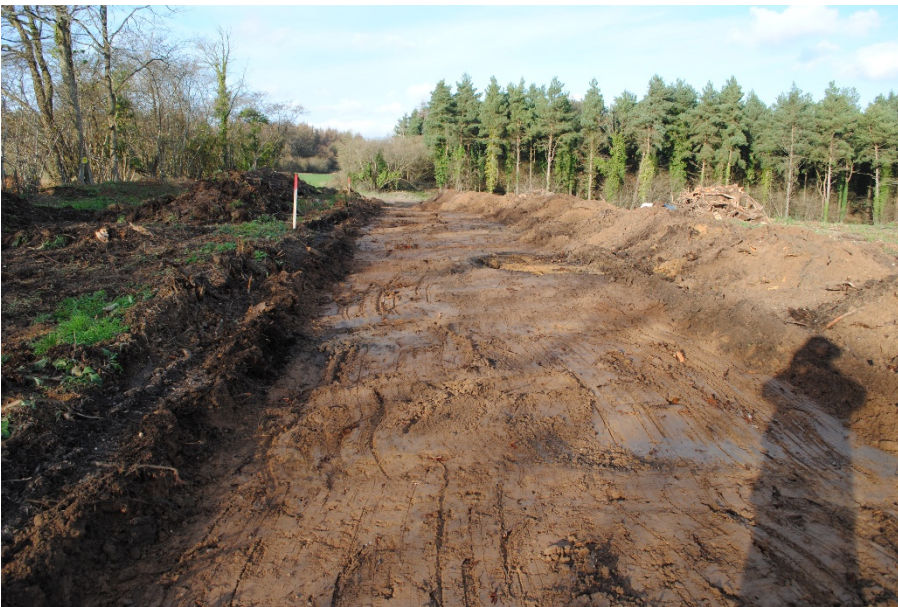
Plate 2: Initial stages of subsoil strip. View from south.
