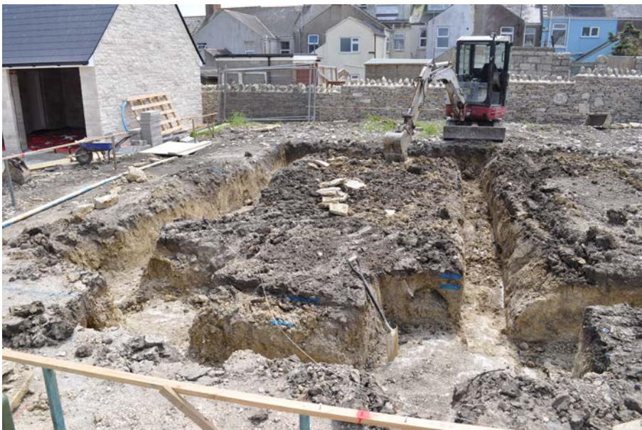
Plate 2: Trench 6 viewed from north.
