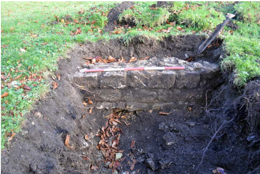
Plate 2: West elevation of Wall 113 in Test Pit 2. 1m scale.
