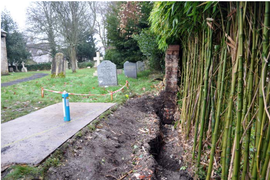
Plate 5: West end of trench showing straight joint at end of surviving churchyard wall.
