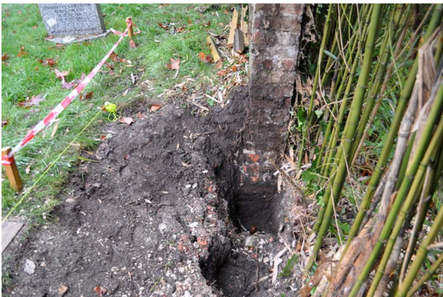
Plate 6: Fence posthole against churchyard wall showing deposits below wall.
