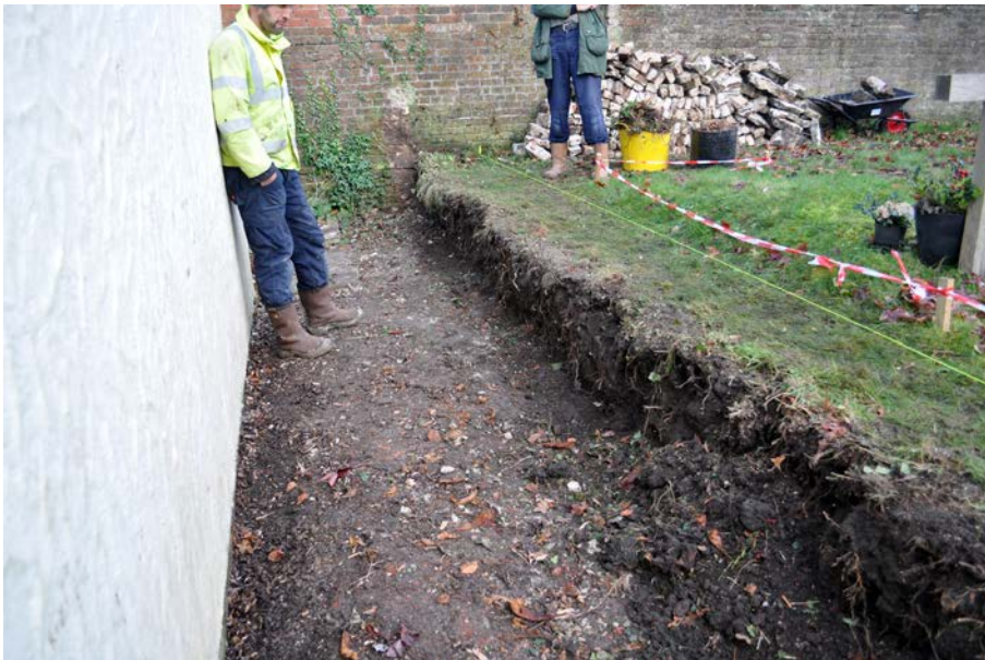
Plate 2: View of east part of area after removal of churchyard wall.
