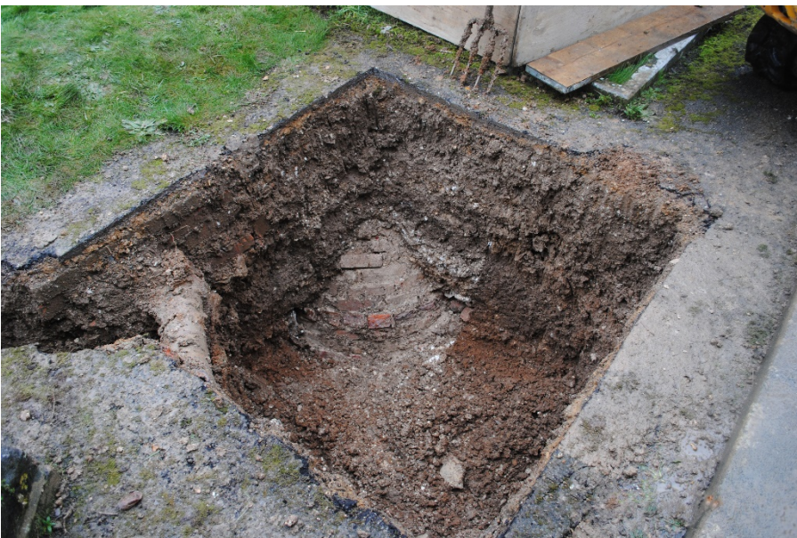
Plate 3: Exposure of corbelled brick structure 106 in construction cut 104. View from west.
