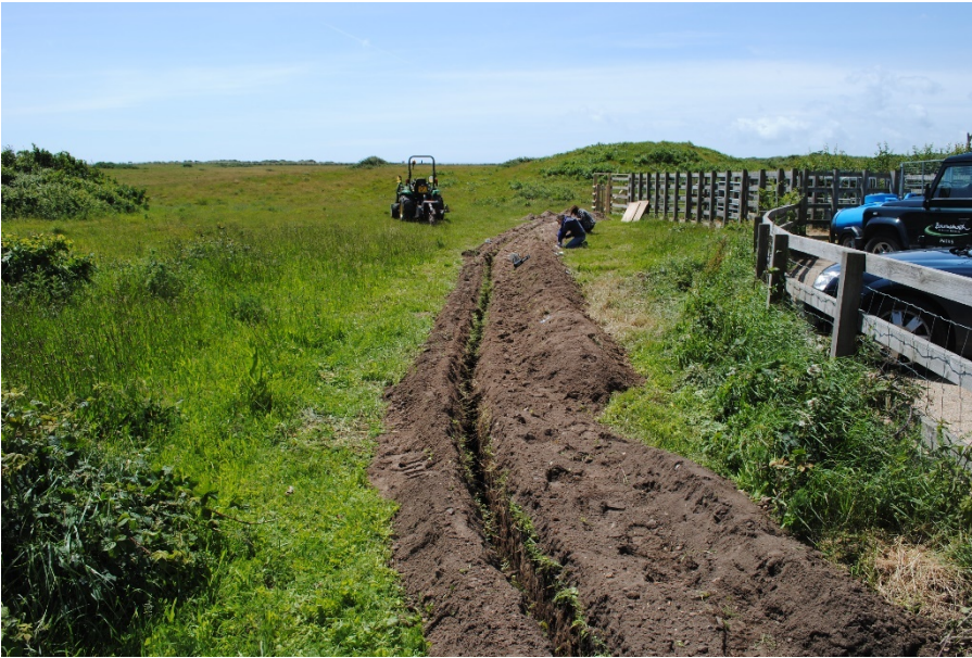
Plate 1: Pipe trench east of the Visitor Centre. View from north.
