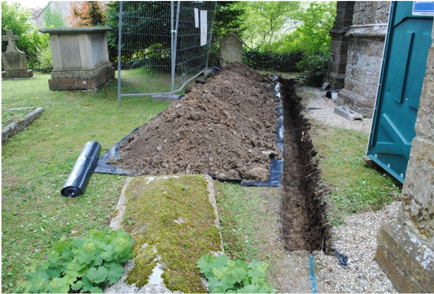
Plate 1: Pipe trench south of Nave and West Tower. View from east.
