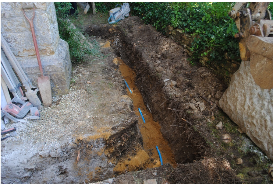
Plate 3: Pipe trench west of West Tower. View from north.
