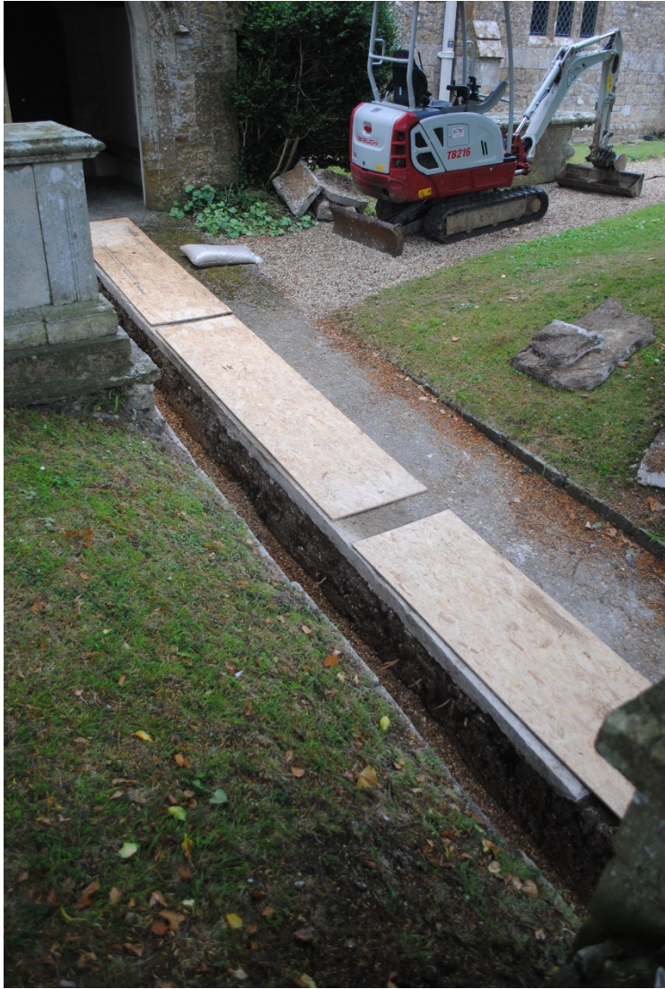
Plate 4: Pipe trench along south path to Nallers Lane. View from south.
