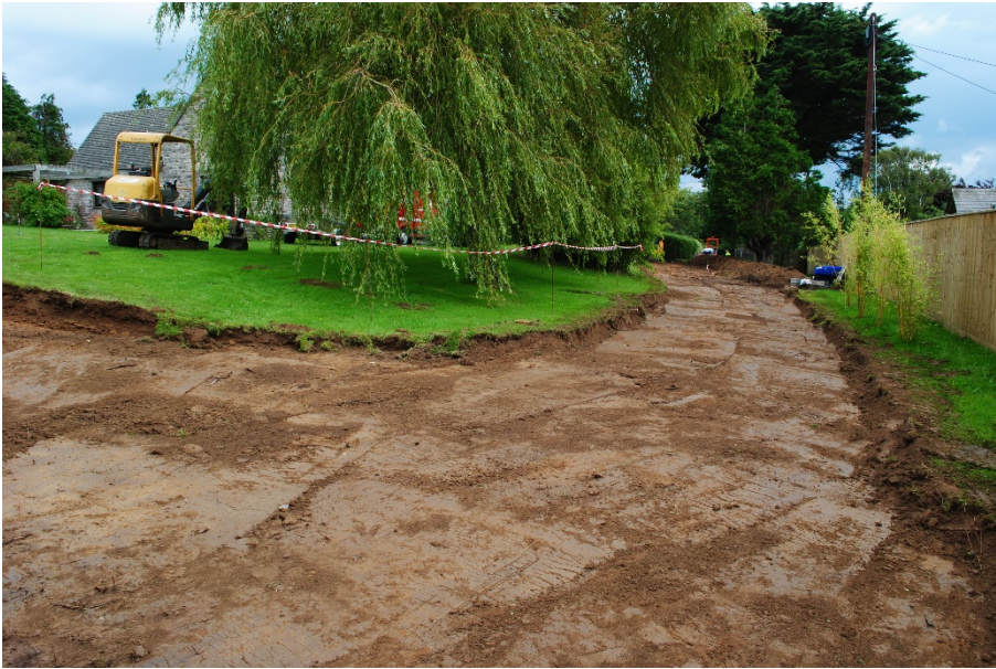
Plate 4: New access route. View from west
