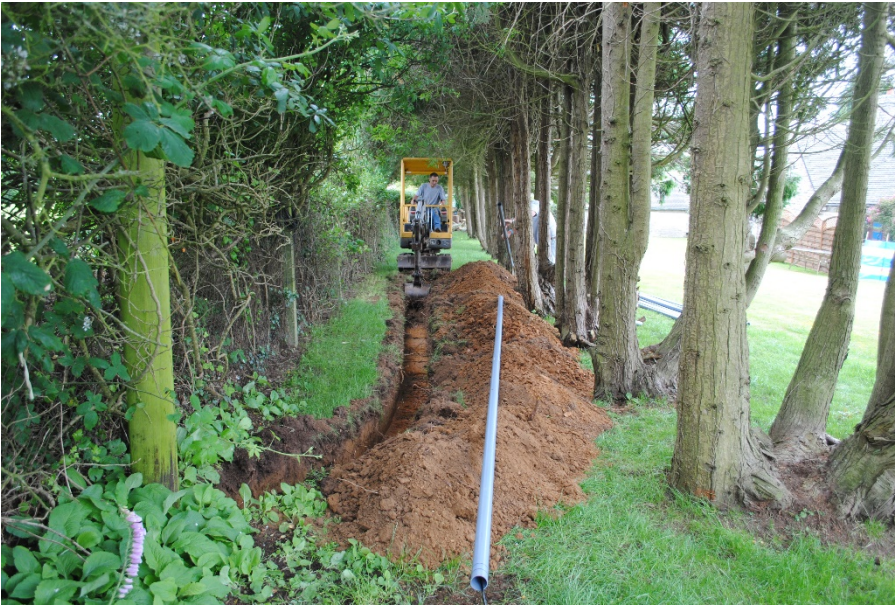
Plate 1: New service trench under excavation. View from west.
