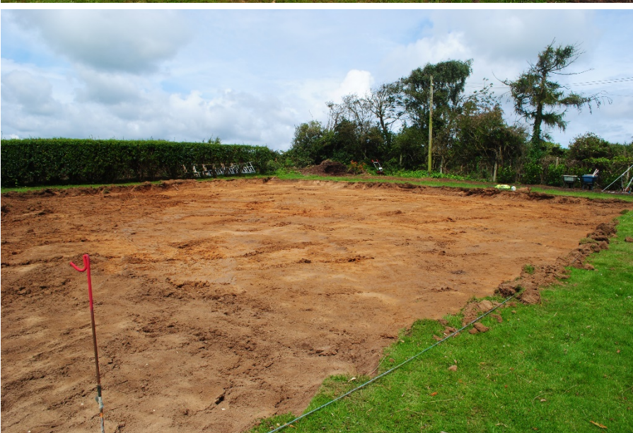
Plate 3: New house footprint area fully topsoil stripped. View from south.
