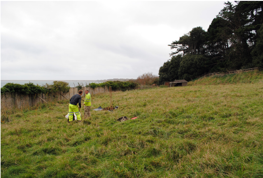
Plate 5: Location of Borehole BH12, looking west.
