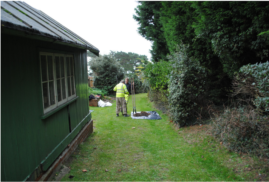
Plate 1: Borehole BH10 during digging of inspection pit, looking south.
