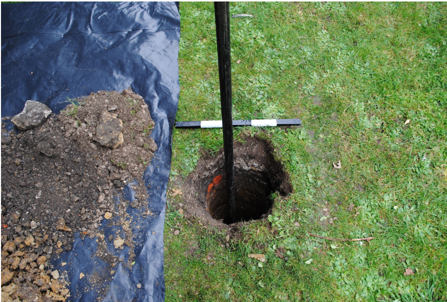
Plate 2: Inspection pit for Borehole BH10, looking north. 0.5m scale.
