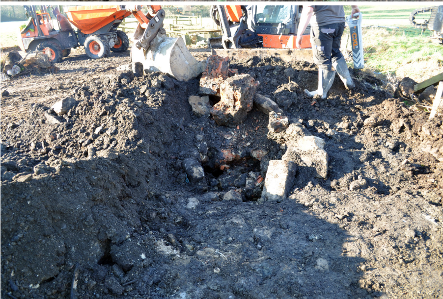
Plate 3: Large rubble infill (216) of former pond on site of new Boiler House.
