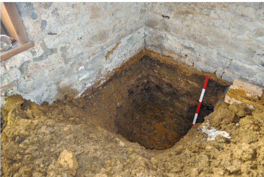
Plate 12: Footings 306 of South Stables exposed in Trench 17, looking south west. 1m scale.
