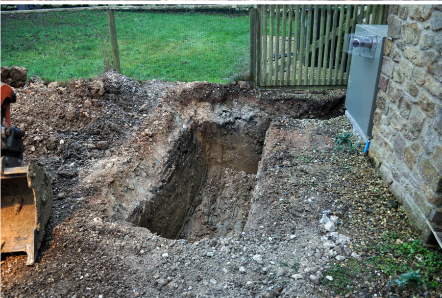
Plate 15: Trench 19 dug in front of Old Rectory Stables, looking east.
