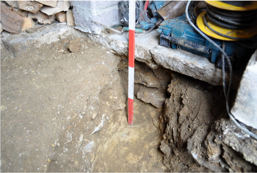
Plate 10: Wall Footing 173 below stone flag floor 175. 1m scale.
