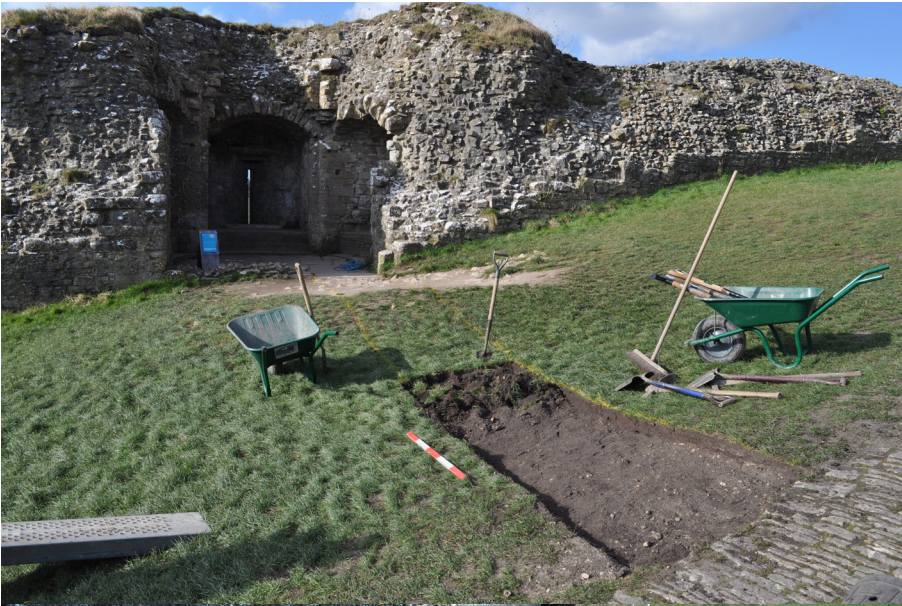
Plate 1: Trench 1 during excavation. View from east. 1m scale.
