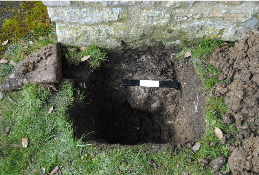
Plate 1: Test Pit 1, showing the rubble footing of the South Porch. View from East. 0.3m scale.
