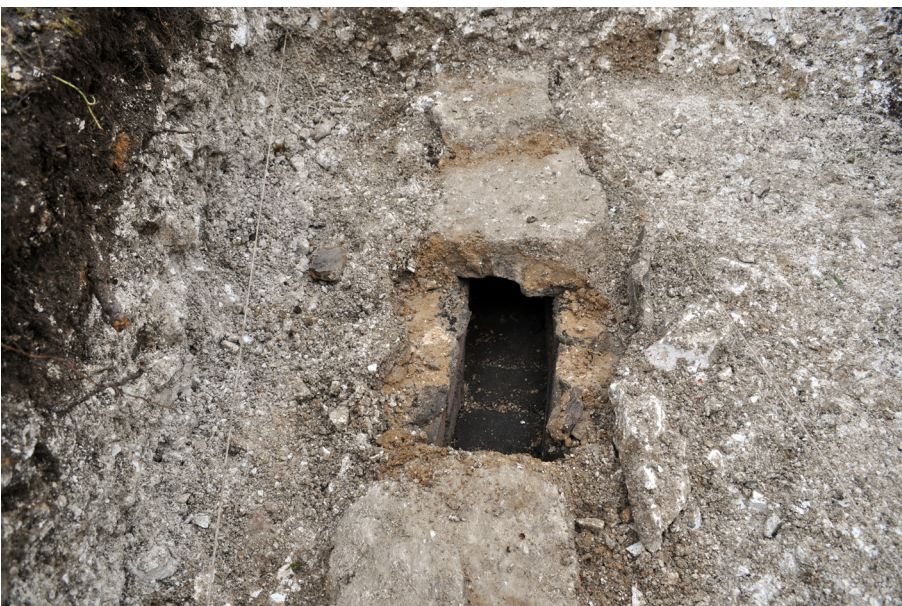
Plate 6: Detail of Drain 305. Viewed from North.
