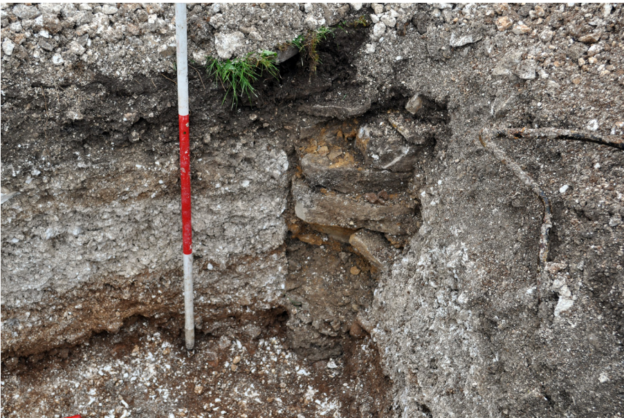
Plate 5: Buttress 202 in north east corner of Trench 2. Viewed from South. 2m scale.
