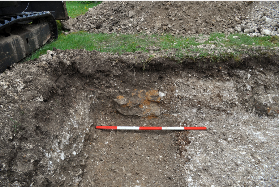
Plate 4: South Wall 308 of the Nave of Christ Church with mortared crushed stone footing 309 below. Viewed from West. 1m scale.
