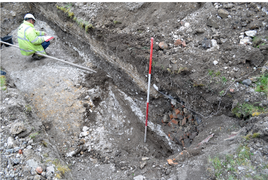
Plate 3: Edge of Outer Ditch 117 of the Roman Town defences in machine sondage at east end of Trench 1. Viewed from West. 2m
