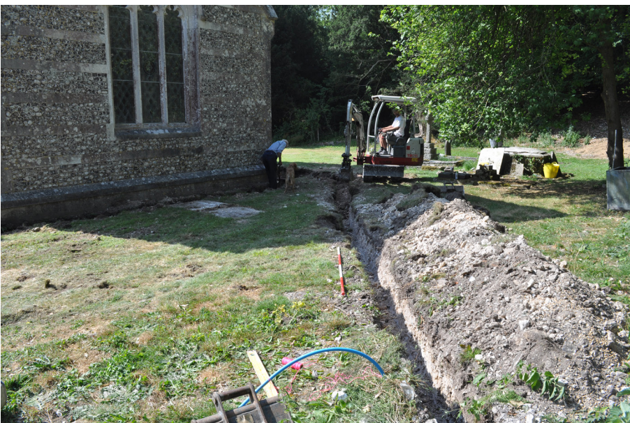
Plate 9: Trench 2 looking North West. 2m scale.
