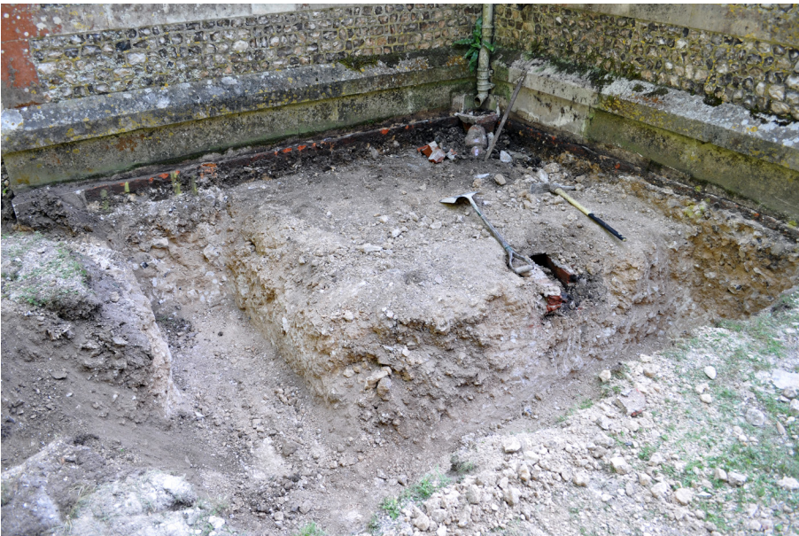
Plate 5: Trench 1 after excavation of new foundation trenches.
