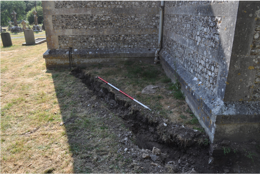
Plate 7: Trench 3 running from South Transept to corner of Chancel. 2m scale.
