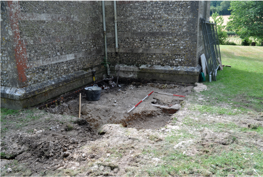
Plate 1: General view of Trench 1, looking South West. 2m scale.
