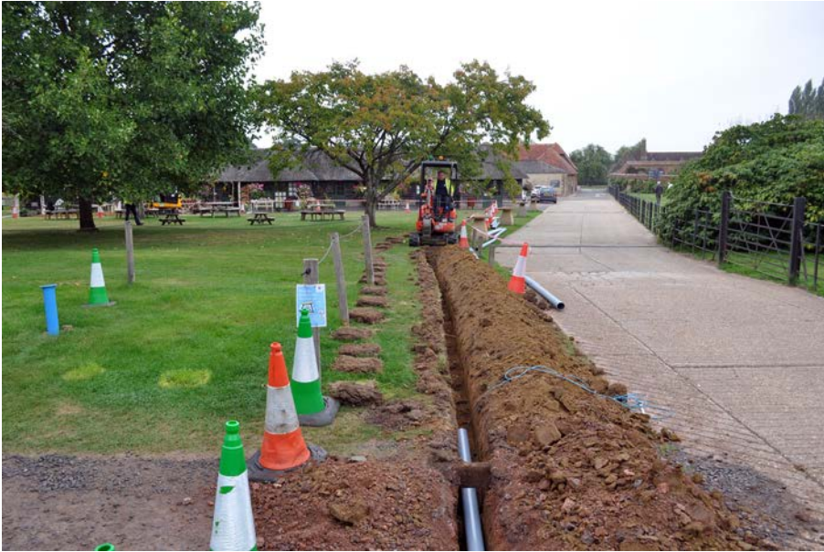
Plate 1: View along trench from south east.
