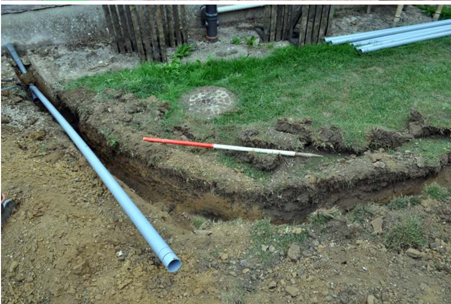
Plate 6: Services disturbance 108, viewed from west. 1m scale.
