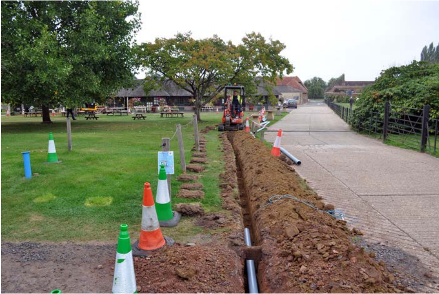
Plate 1: View along trench from south east.
