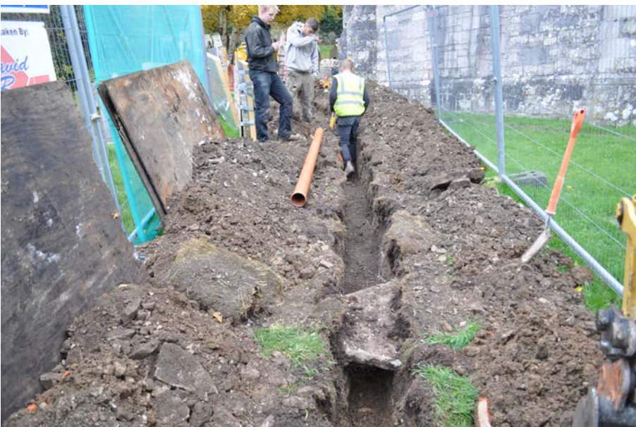
Plate 6: Ledger slab 110 (broken parts removed), looking south.
