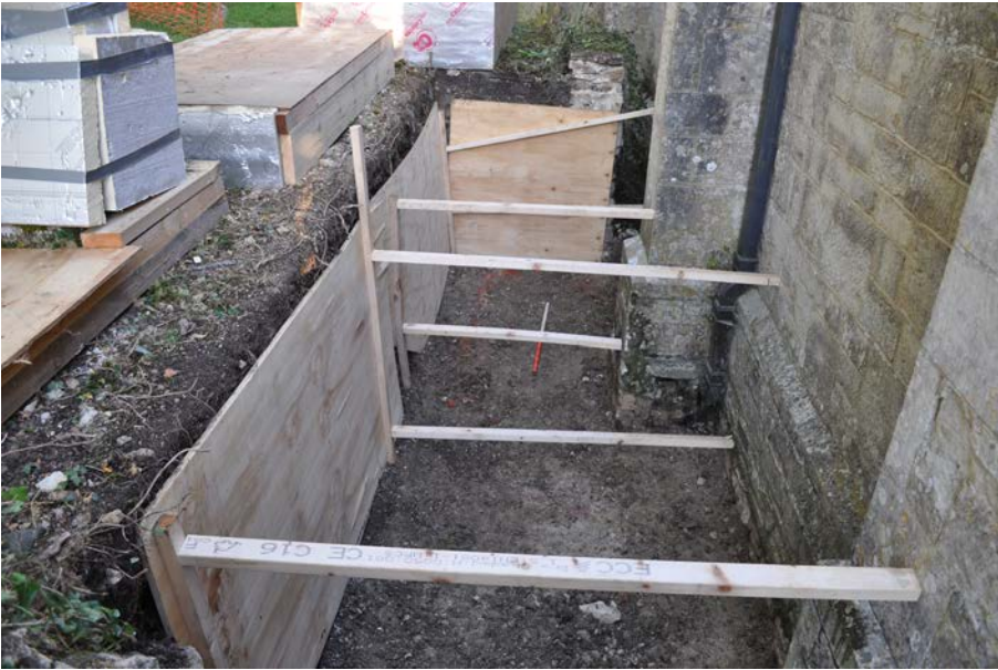
Plate 1: Area of new extension after clearance, looking west.
