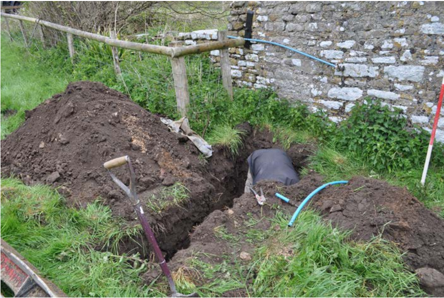
Plate 7: General view of Trench 3 after excavation, looking north.
